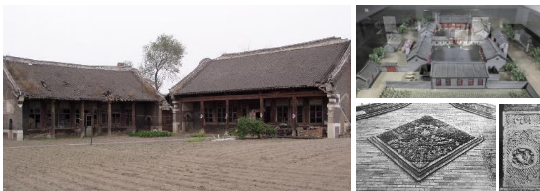
Current state of the building and architectural details
