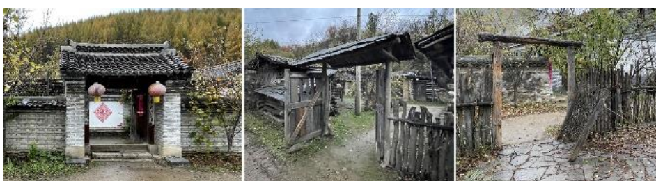
Fig 12. House-style gate; wooden board gate; pole gate (Photographed and drawn by Zhao Liangyu)
