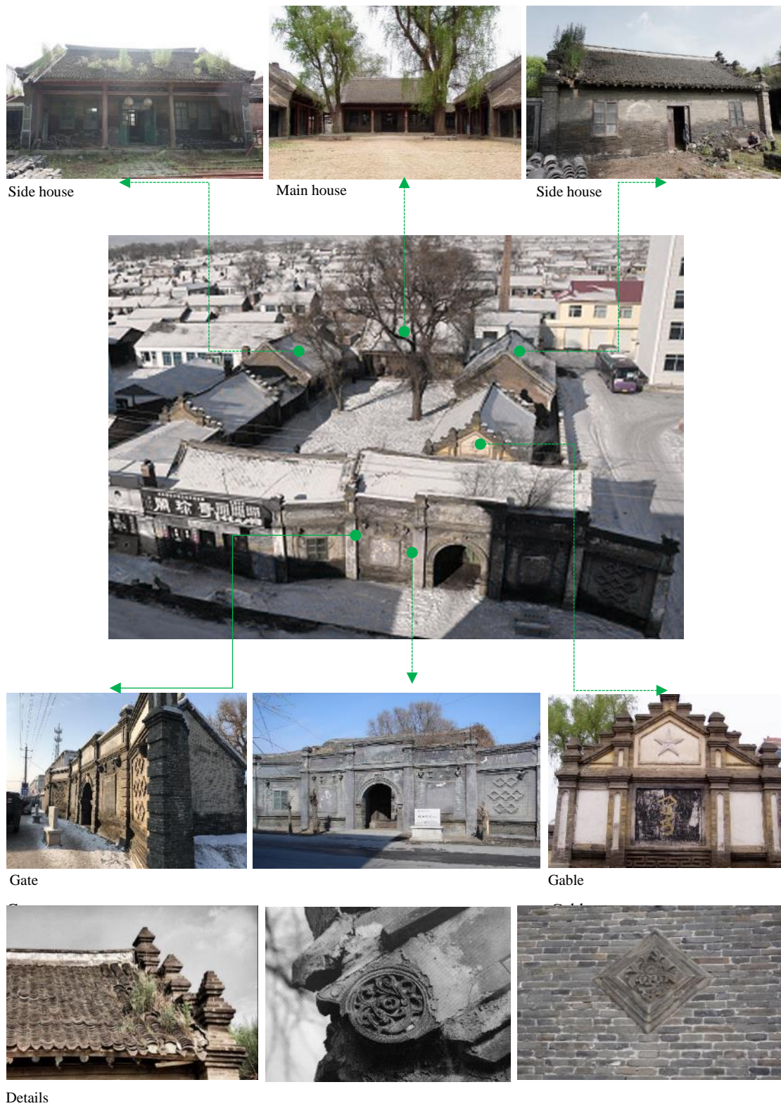
Fig 81. The original historical appearance of Historic building-Kui Mansion (Photographed by Zhao Liangyu)
