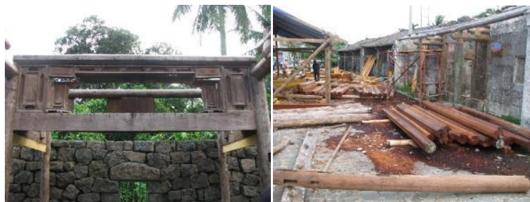
Fig 26. Restoration of the Confucius Hall
