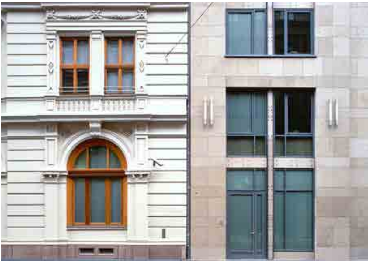
Raiffeisen Bank headquarters, Budapest Széchenyi Emebankment - Akadémia Street (architect: Finta Studio)
