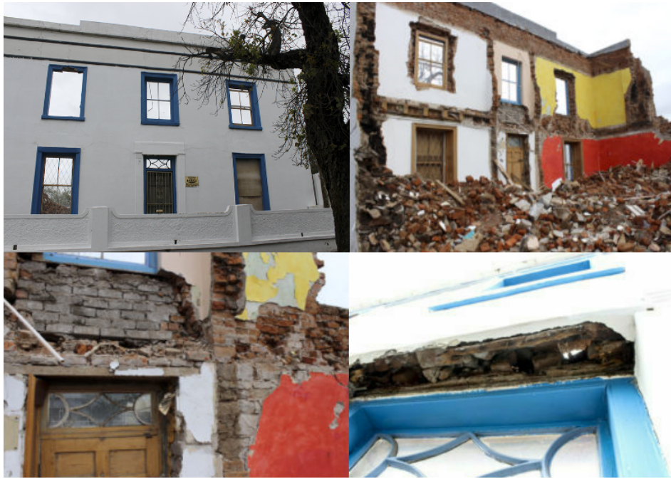
Figure 7. Assessment of construction of the historic property at 68 Bathurst Street
