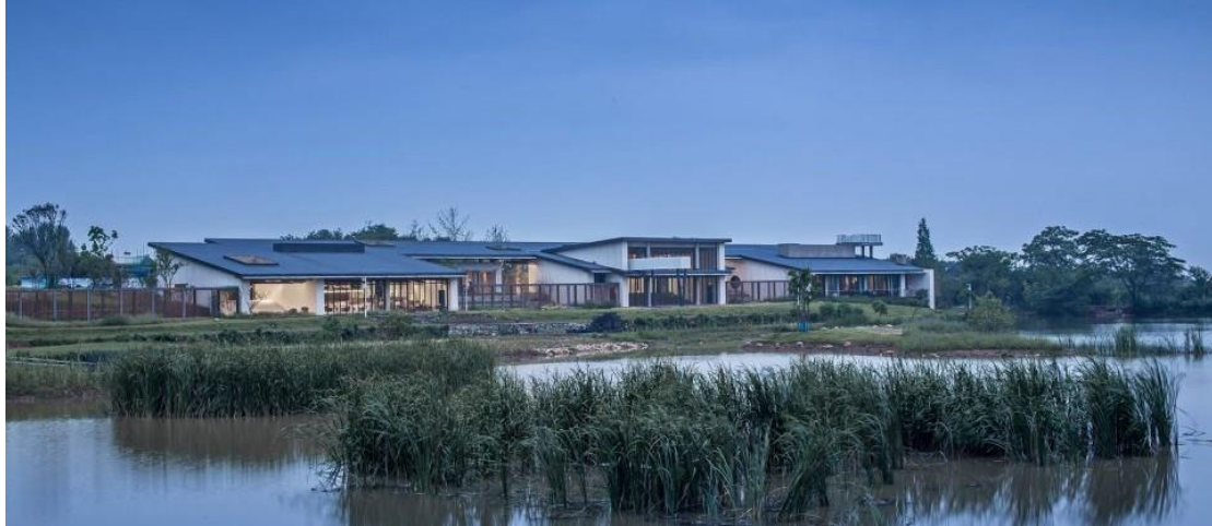
The Culture Reception Hall in Tingrui Town, China (Photographed by UAO Design Company)
