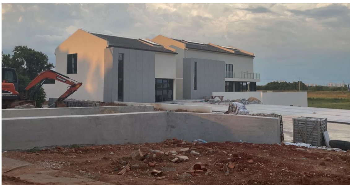
Fig. 90 On-site photo of Tourist Reception Center (Photographed by author)
