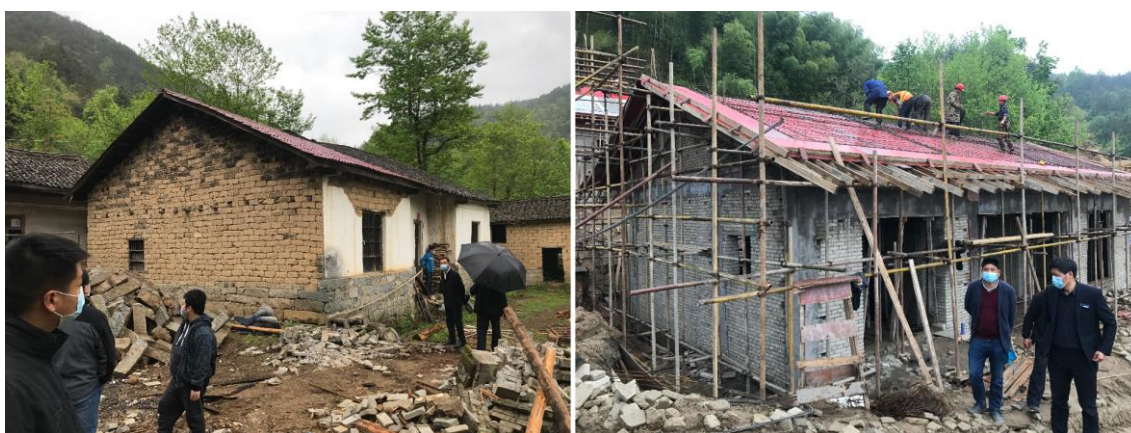
Fig. 105 Original Building Photos and Construction Site Photos (Photographed by author)
