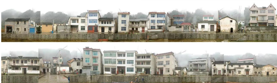
Fig. 29 Architectural Facades in Wencun Village (36kr.com)
