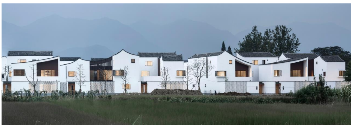
Fig. 38 Relocation Houses in Dongziguan Village, Hangzhou, China (www.archiposition.com)
