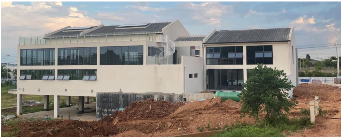
Fig. 93 On-Site Photo of Tourist Reception Center (Photographed by author)
