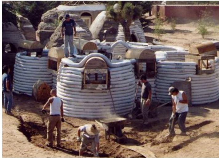
Figure 64: A sample of the sandbag house in California designed by Nader Khalili source: [111]
