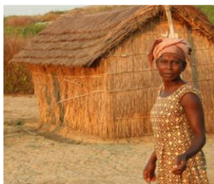
Figure 23: the wooden gable frame shelter. Source: [25]
