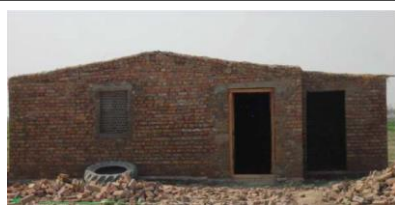
Figure 17: A one room shelter by UNHCR
