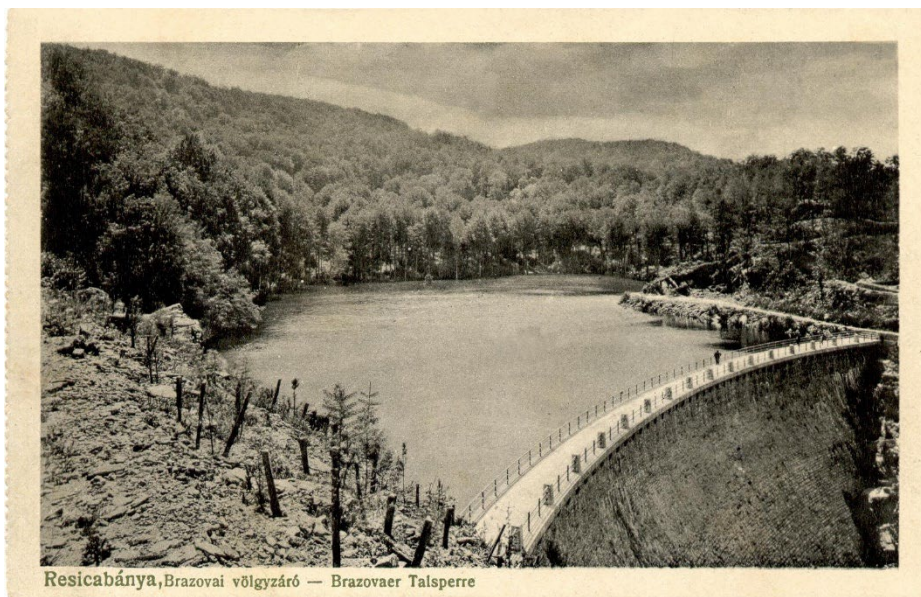
Figure 9 The water reservoir in Breazov; Kulhanek collection
