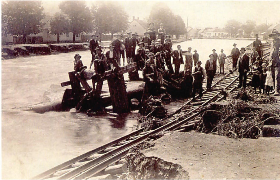
Figure 11 Flooded highway and railway track, 1912; Kulhanek collection
