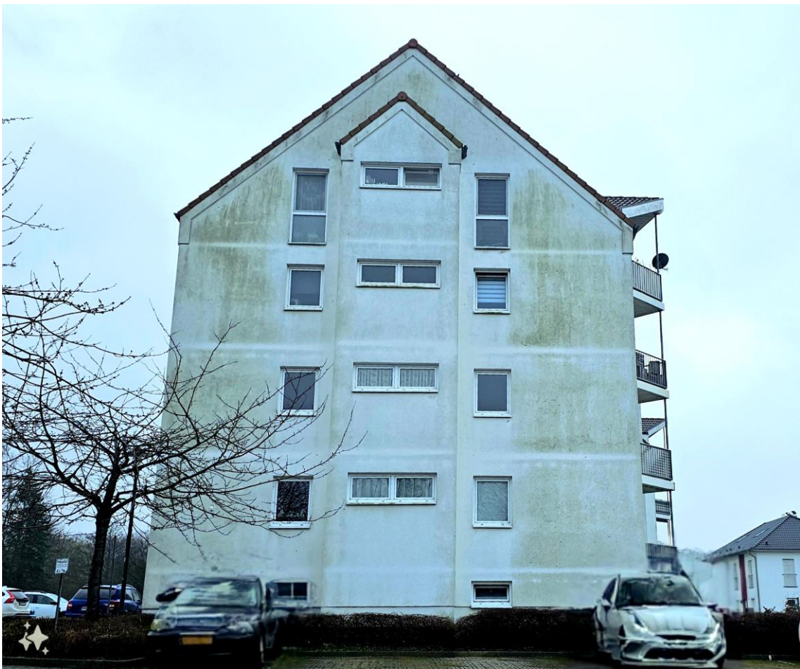
Figure 1: North gable near Wismar/Germany after 7 years of renovation (Photo: Author)
