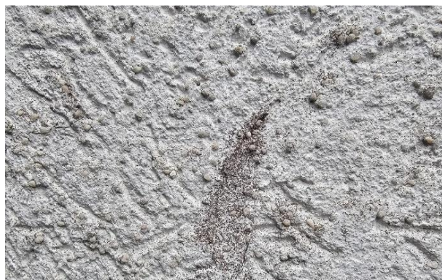
Figure 13: ETICS with algae infestation starting around marble grains
