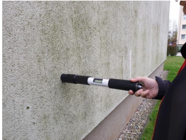
Figure 5: Application of Benthos Torch at building facade in Wismar/Germany [53]
