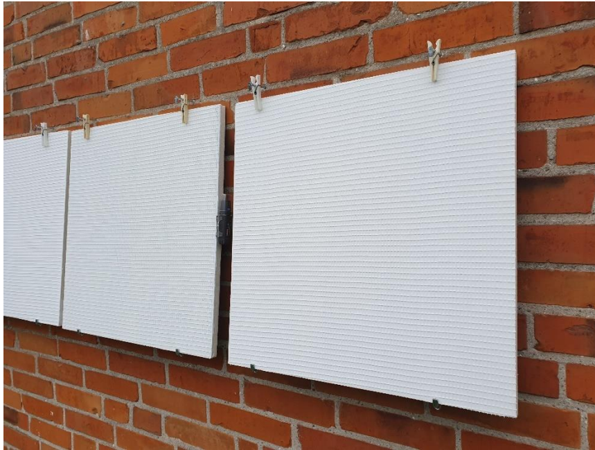
Figure 53: Mounting and fixing of samples at the brick wall north gable
