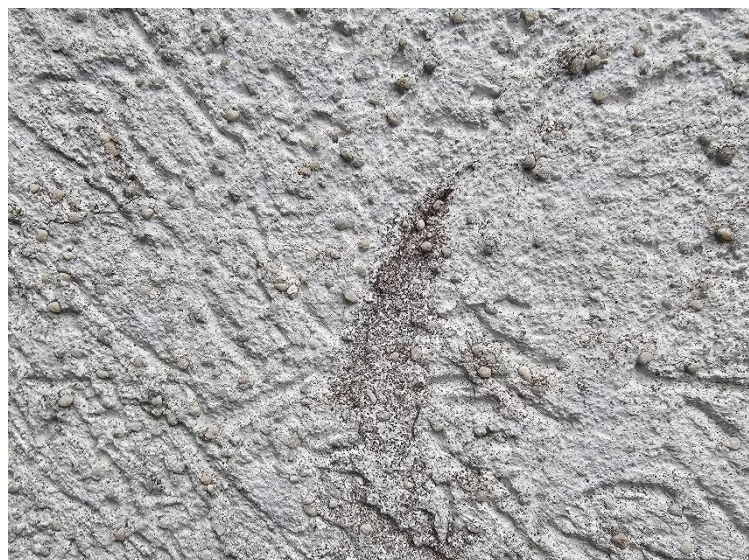
Figure 43: ETICS with algae infestation starting around marble grains
