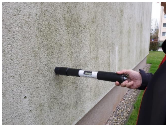
Figure 15: Application of BenthosTorch at building facade in Wismar/Germany
