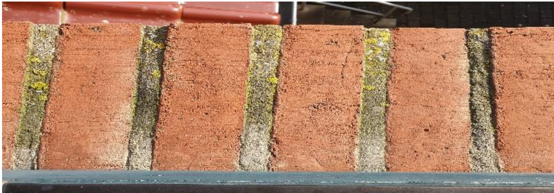
Figure 6: Biofilm formation on 13-clinker brine bank (detail picture)
