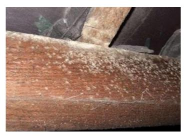
Figure 1. Fungai decay on timber column [The Constructor, 2021]
