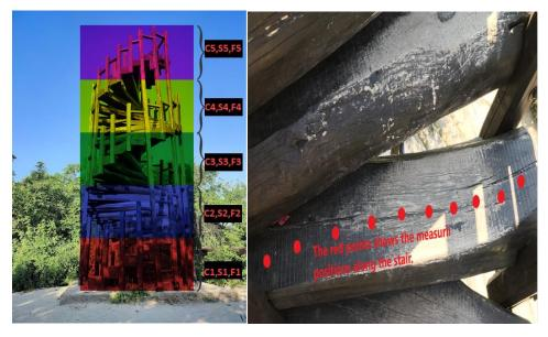
Figure 34. On-site measurement process in the Makovecz Imre lookout tower [own photo]
