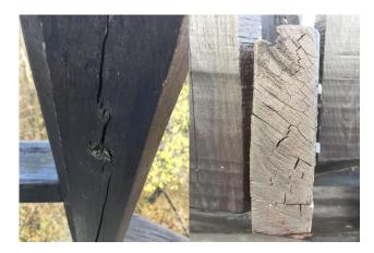
Figure 33. Cracks in the Makovecz Imre lookout tower [own photo]
