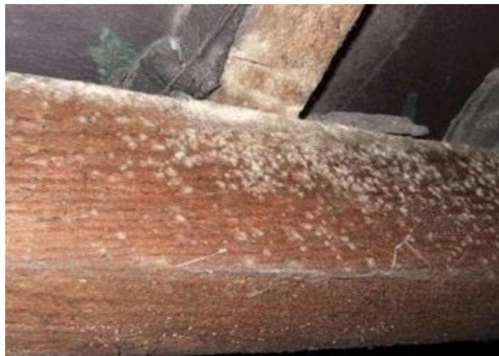
*Figure 1. Fungai decay on timber column [The Constructor, 2021]*
