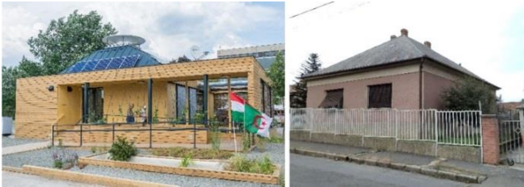
Figure 4.1. The refurbishment design project from SDE19 competition (left), a typical ‘Cube house’ in Pécs, Hungary (right)
