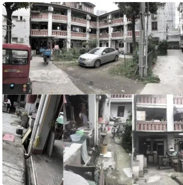
Fig.32 Situation before renovation
