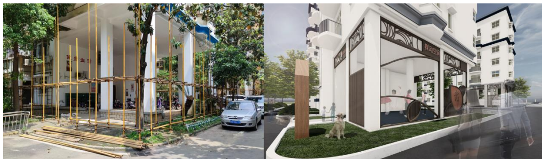
Fig.73 Opening space rendering pictures and physical picture (Source: Drawing by the author)
