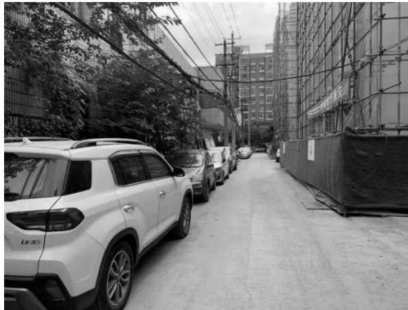
Fig.83 Traffic situation (Source: photo by the author)
