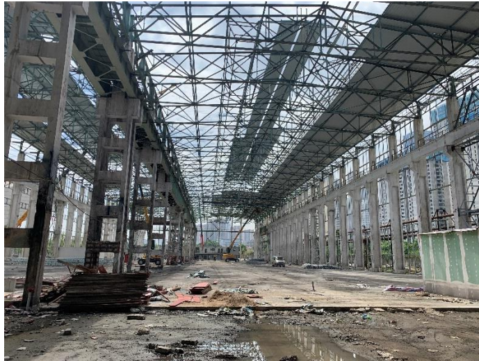
Fig.90 Site situation before renewal (Source: photo by author)
