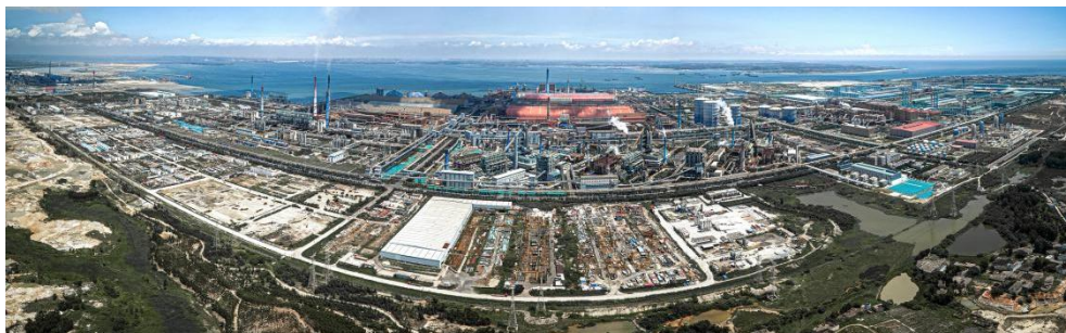
Fig. 4-2. Aerial photography of Zhanjiang Steel Factory (Source: photo by GDAD)
