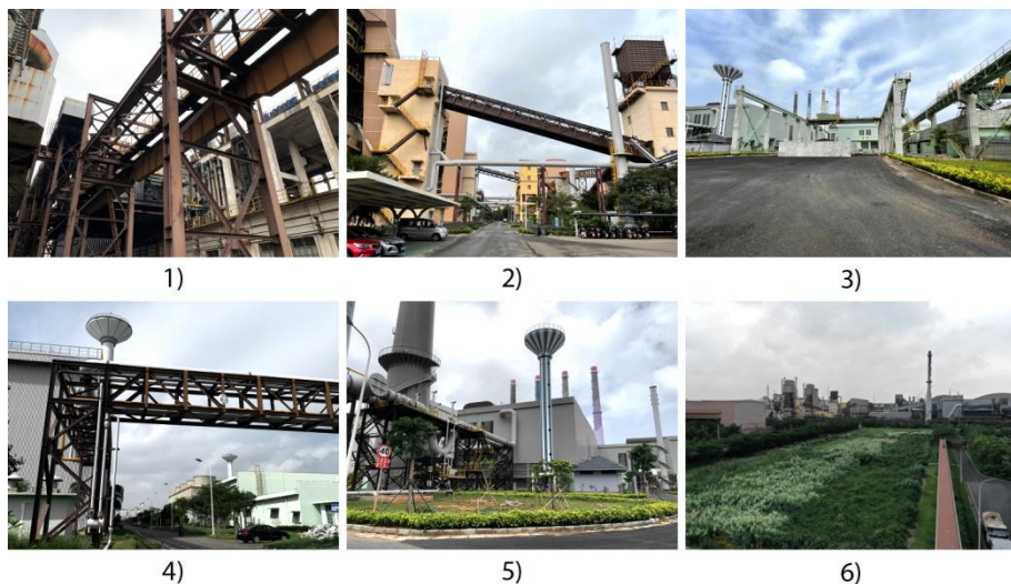
Fig. 4-4. 1) Iron plant, 2) steel plant, 3) hot rolling plant, 4) cold rolling plant, thick plate plant, 5) water control center (Source: drawn by author)
