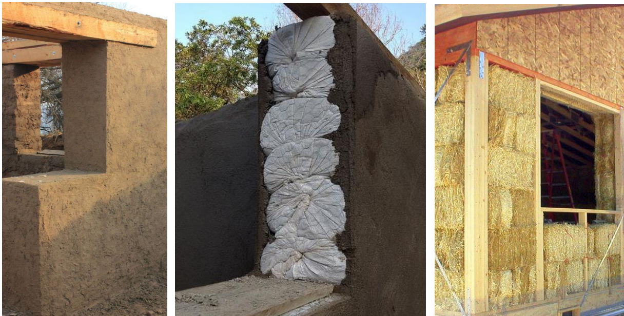
Figure 2-3 Cob, earthbags and straw bales construction techniques
