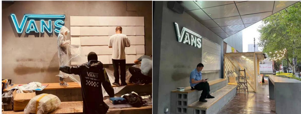
Figure 86. Construction process (Source: Photographed by Jin He)
