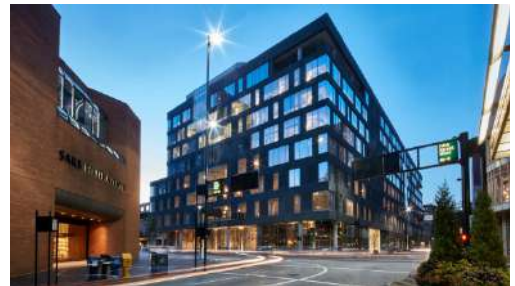
Figure 88: 84.51 Centre office building, designed by Gensler
