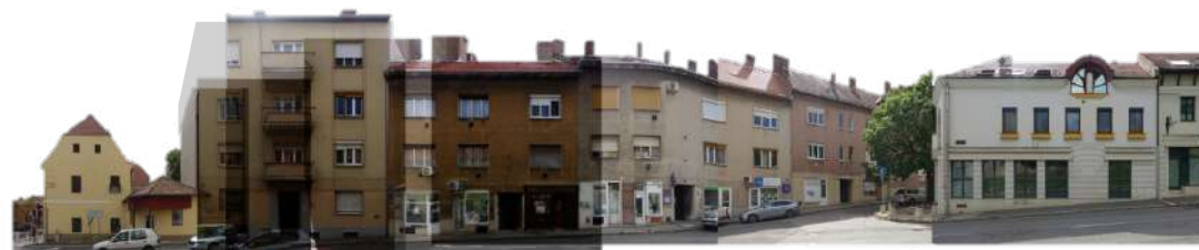
Alkotmány Street Elevation – West sidewalk →
