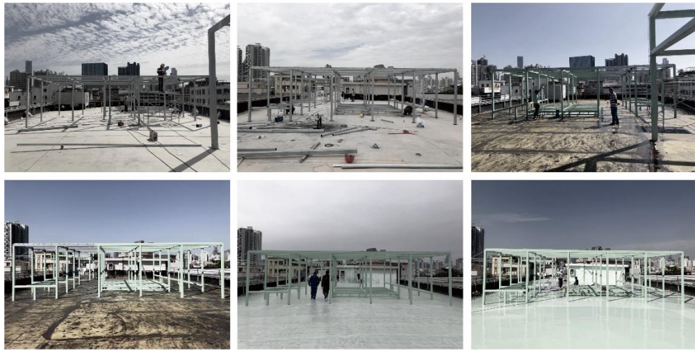
Modular unit construction process
