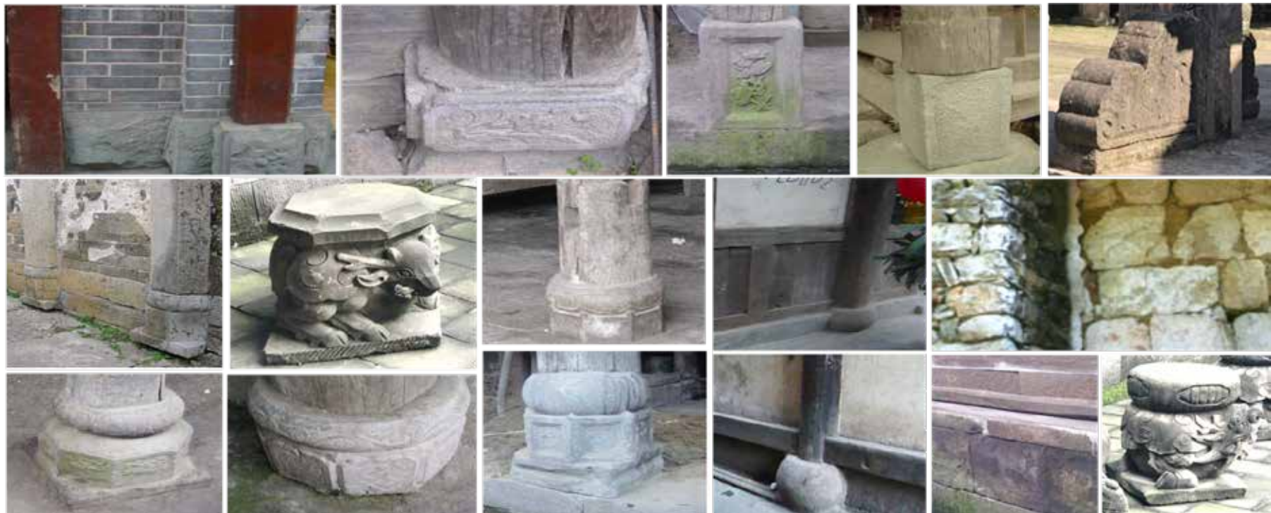
Fig 4.33: The basis of Vernacular Architecture in Chongqing(source: photo by author)
