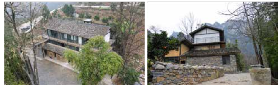
Fig 5.17: Building 1 under construction (source: photo by author)
