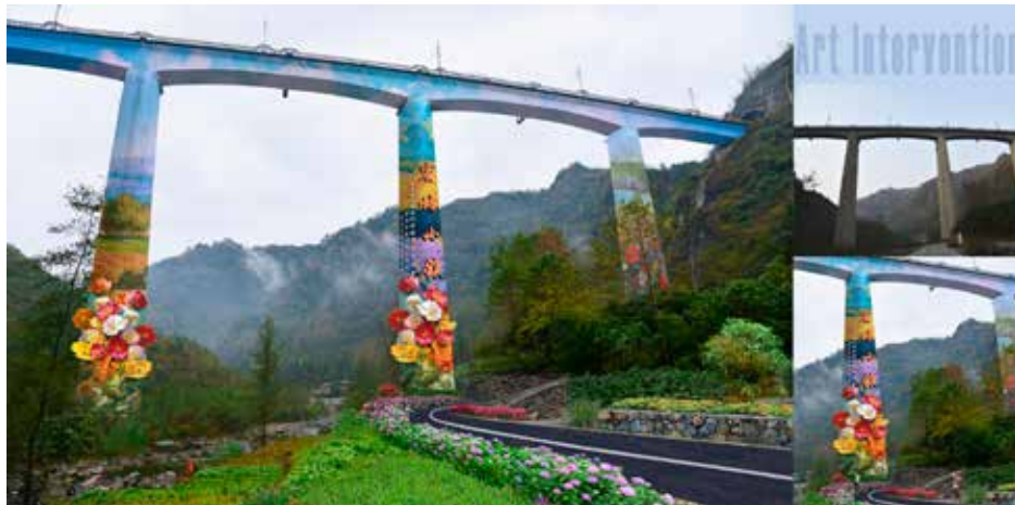
Fig 5.38: Viaduct columns designed with artistic techniques (source: drawing by author )
