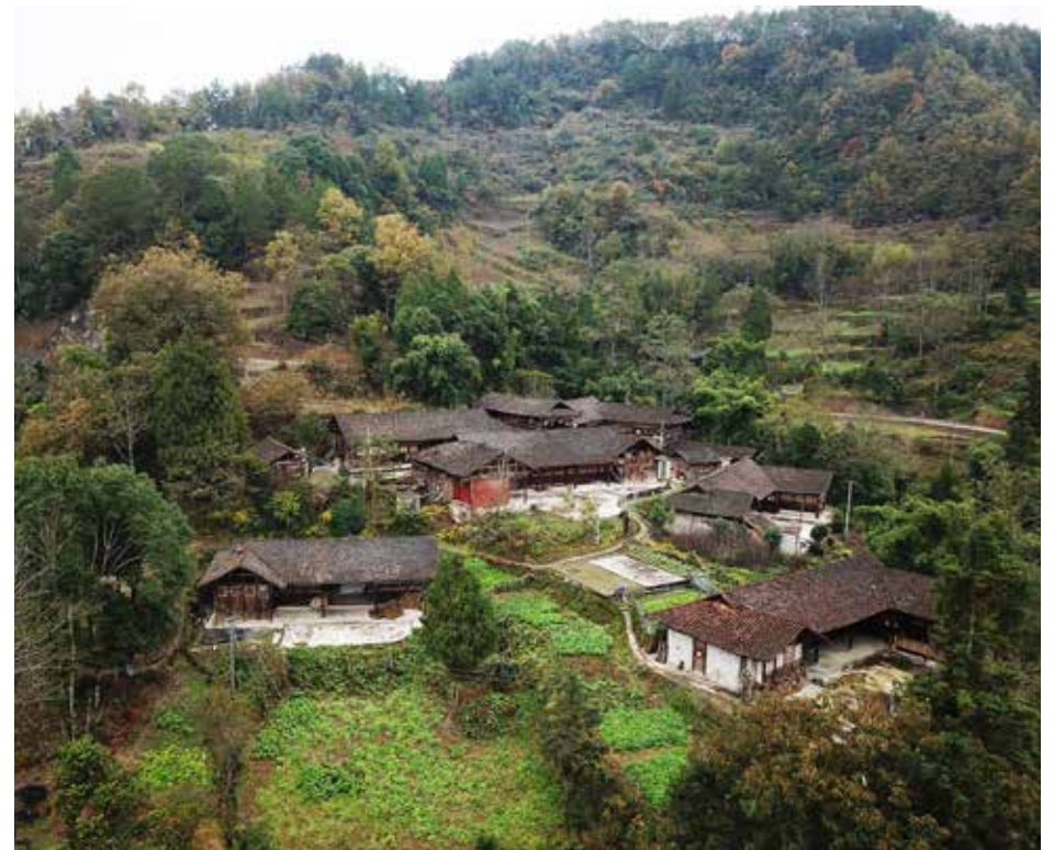
Fig 4.9: Vernacular architecture blends into nature(source:photo by author)
