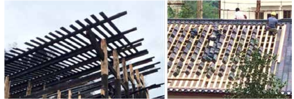
Fig 4.29: The rafter and purline of Vernacular roof (source: photo by author)
