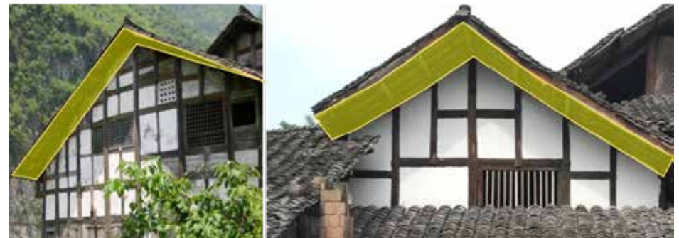
Fig 4.26: Gable roof avoid the erosion of the wall (source: drawing by author)
