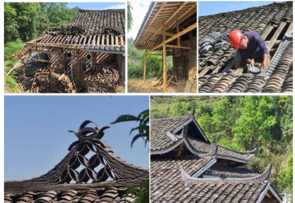
Fig 5.31: Traditional village under construction (source: photo by author)
