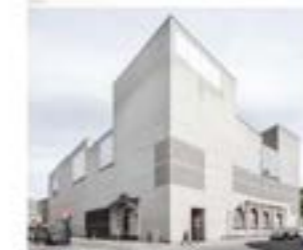
From the ruins of a late-Gothic church to the new Kolumba Museum in Cologne, Germany.
