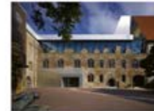
The Moritzburg Museum in Halle, Germany, is an example of a conversion from a semi-ruined roofless castle to a folding structural platform with the addition of a new roof and upper stories.
