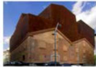
Casa Forum museum in Madrid was transformed from a former power plant.
