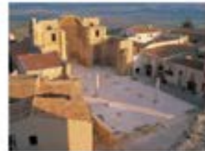
The conversion of the earthquake-devastated 17th-century church (Chiesa Madre) in Salerno, Italy, into a new urban plaza, dictates the addition of a new floor, circulation, structural improvements, and new lighting.
