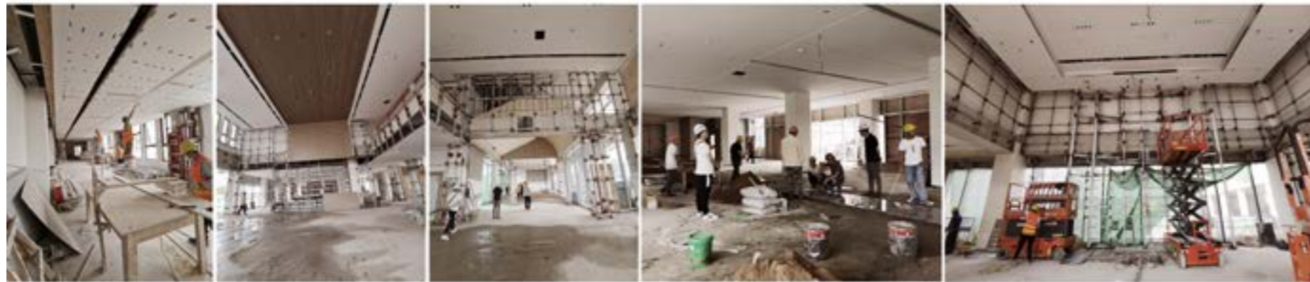
Finishing work stage
