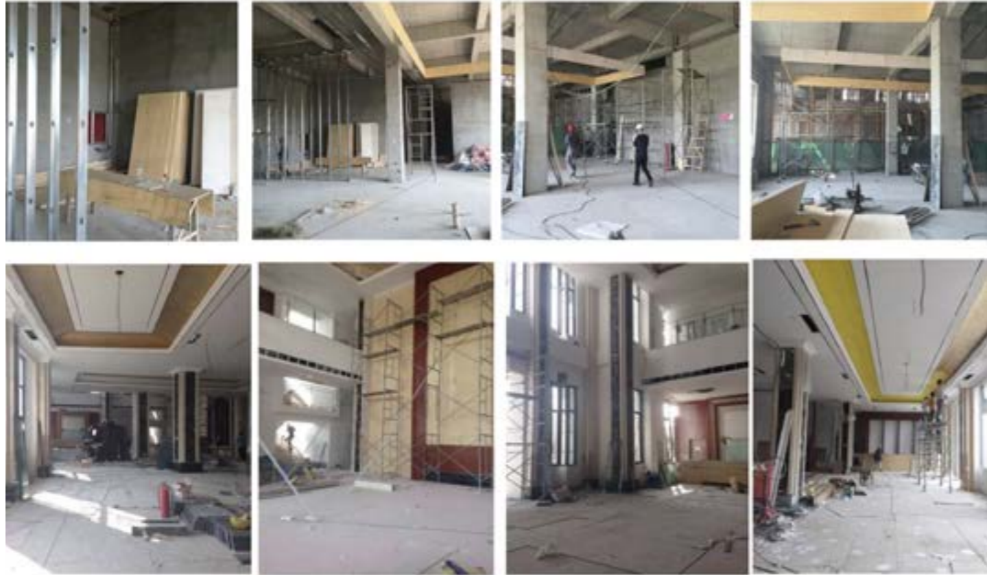
Site of the construction process
