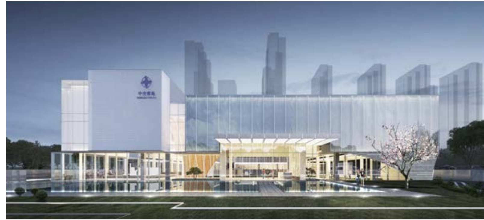
Front elevation of building
