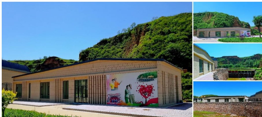
Fig. 37. Real scene of Hougou New Village Day Care Center for the elderly. (Source: Photo & designed by CAO Hui, 2019-2020)
