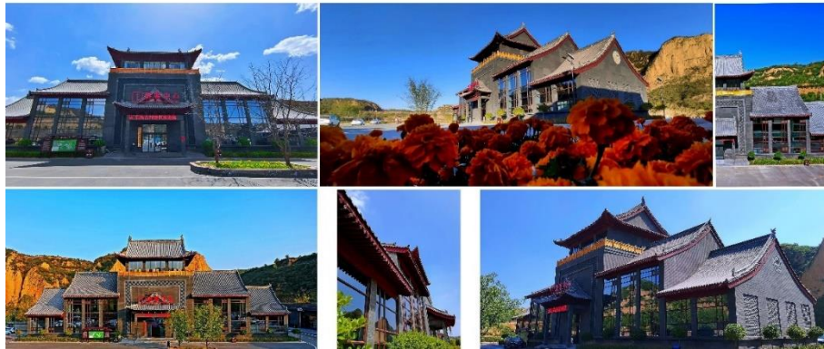
Fig. 44. Facade decoration of Chinese folk Cultural Heritage Rescue Project memorial Hall. (Source: Photo by CAO Hui, 2021)
