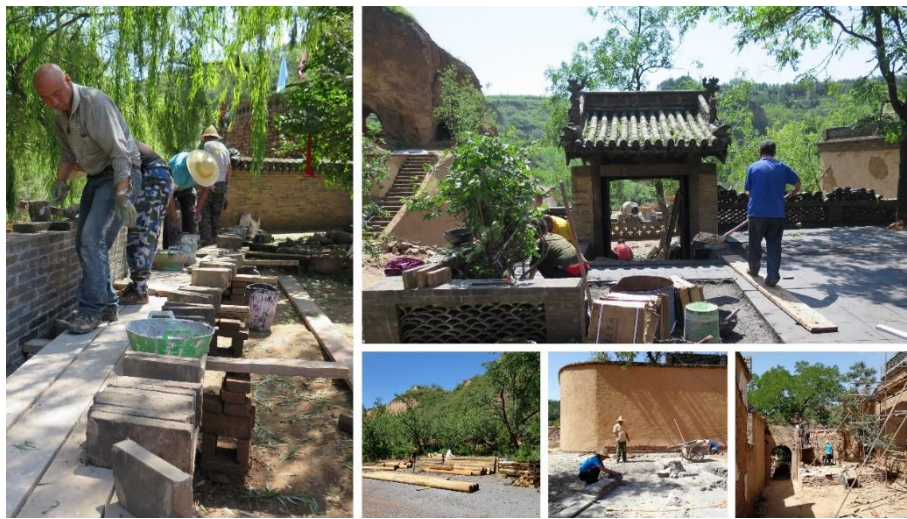
Fig. 66. Restoration process of Hougou Ancient Village.
