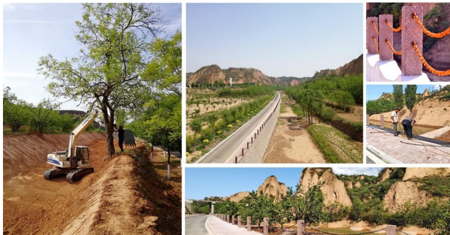
Fig. 55. Longmen River - Waterfront landscape reconstruction project. (Source: Photo by CAO Hui, 2021)
