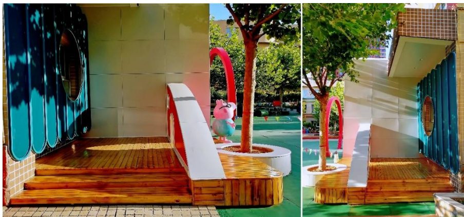
Fig. 106. Real scene of outdoor interactive area of teaching building of Jinzhong No.1 Kindergarten A.
