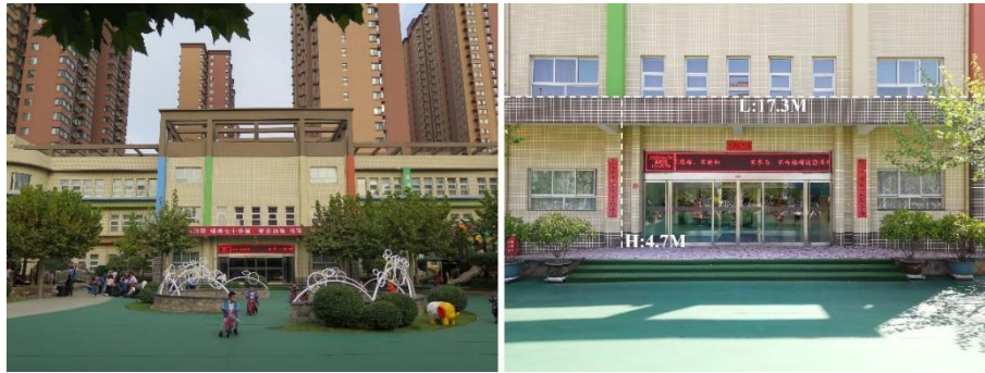
Fig. 95. Status quo of entrance area of teaching building.
