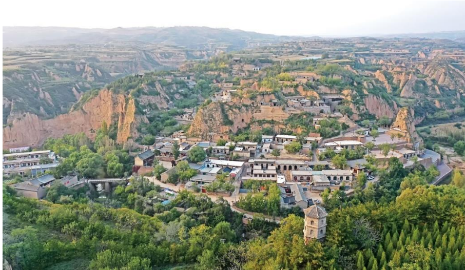
Fig. 71. A panoramic view of Hougou Ancient Village under restoration. (Source: Photo by WANG Yonggang, 2021)
