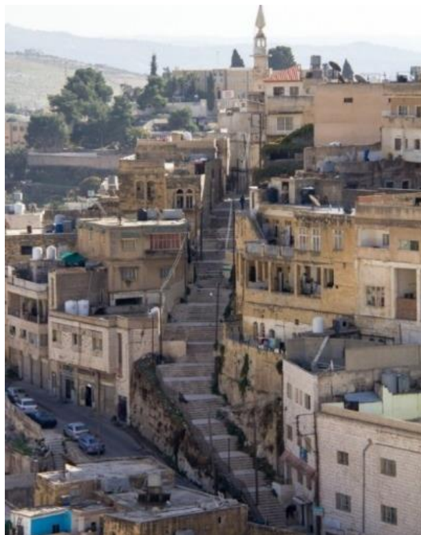
Figure 5.5 B: Salt City stairs
