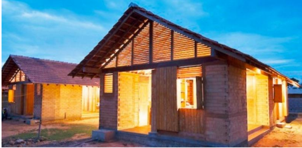
Figure 14. Shigeru Ban is a disaster relief shelter.
