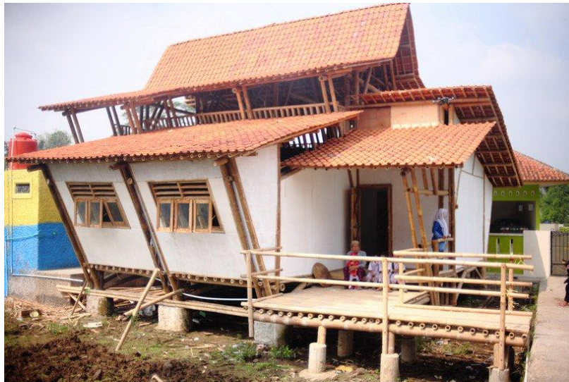
Figure 28. Bamboo Kindergarten House.
