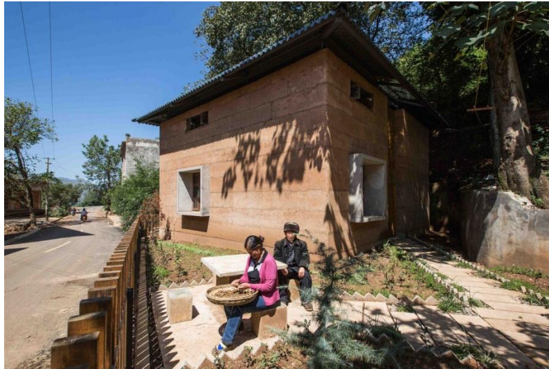
Figure 18. Guangming Village for a Post-Earthquake Reconstruction Project.
