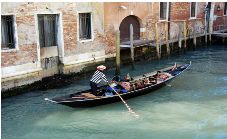
Figure 1: Rising humidity in masonry buildings in Venice (source: www.passengeronearth.com )
