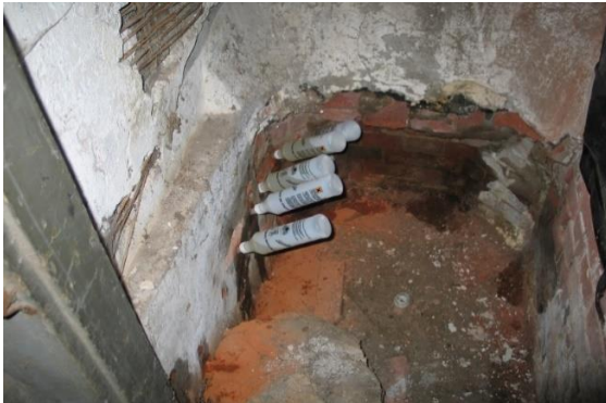
Figure 2: Pressureless injection of injection agent in masonry (source: Dahlberg Institute)
