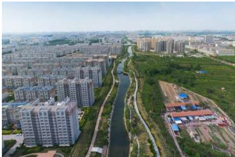
Fig 5-51 Baisha River under construction
