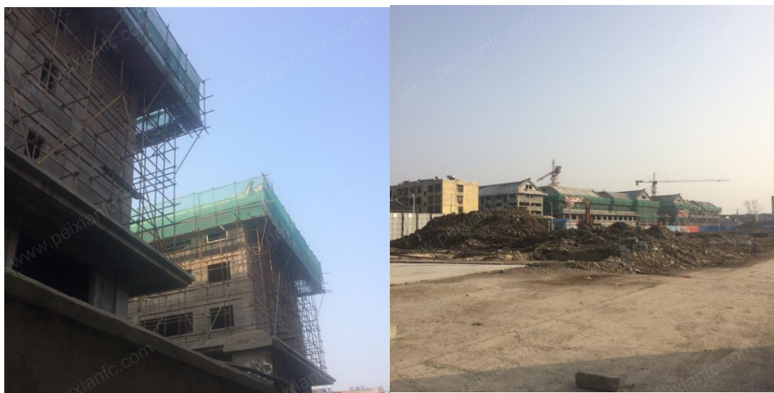
Fig.6.2.9 Actual construction process picture
