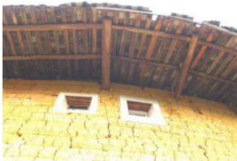
Fig.3.3.2 Fujian Tulou Real Picture of the eaves.
