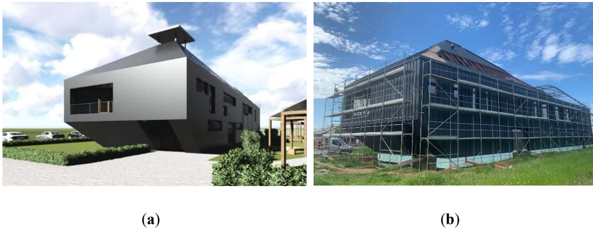
Figure 19. (a) Design visualization rendering and (b) the final building under construction.
