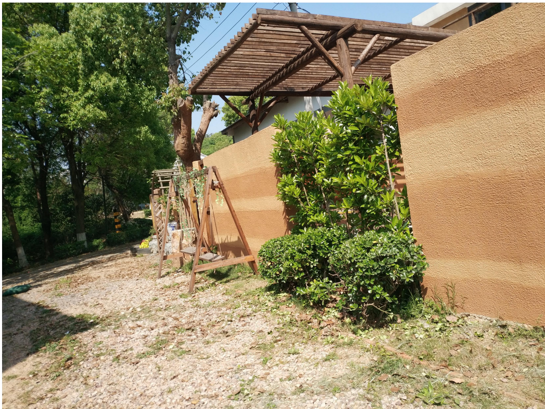
Building C fence(Source: photographed by the author)
