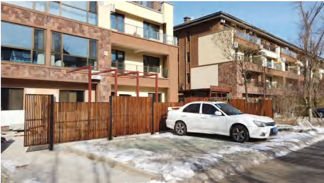
Construction Site Photo, January 2020
