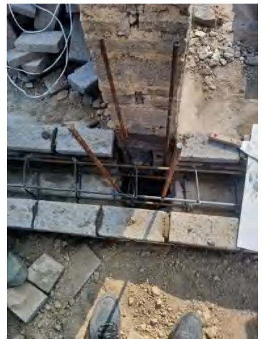
Structural Reinforcement, December 2021
