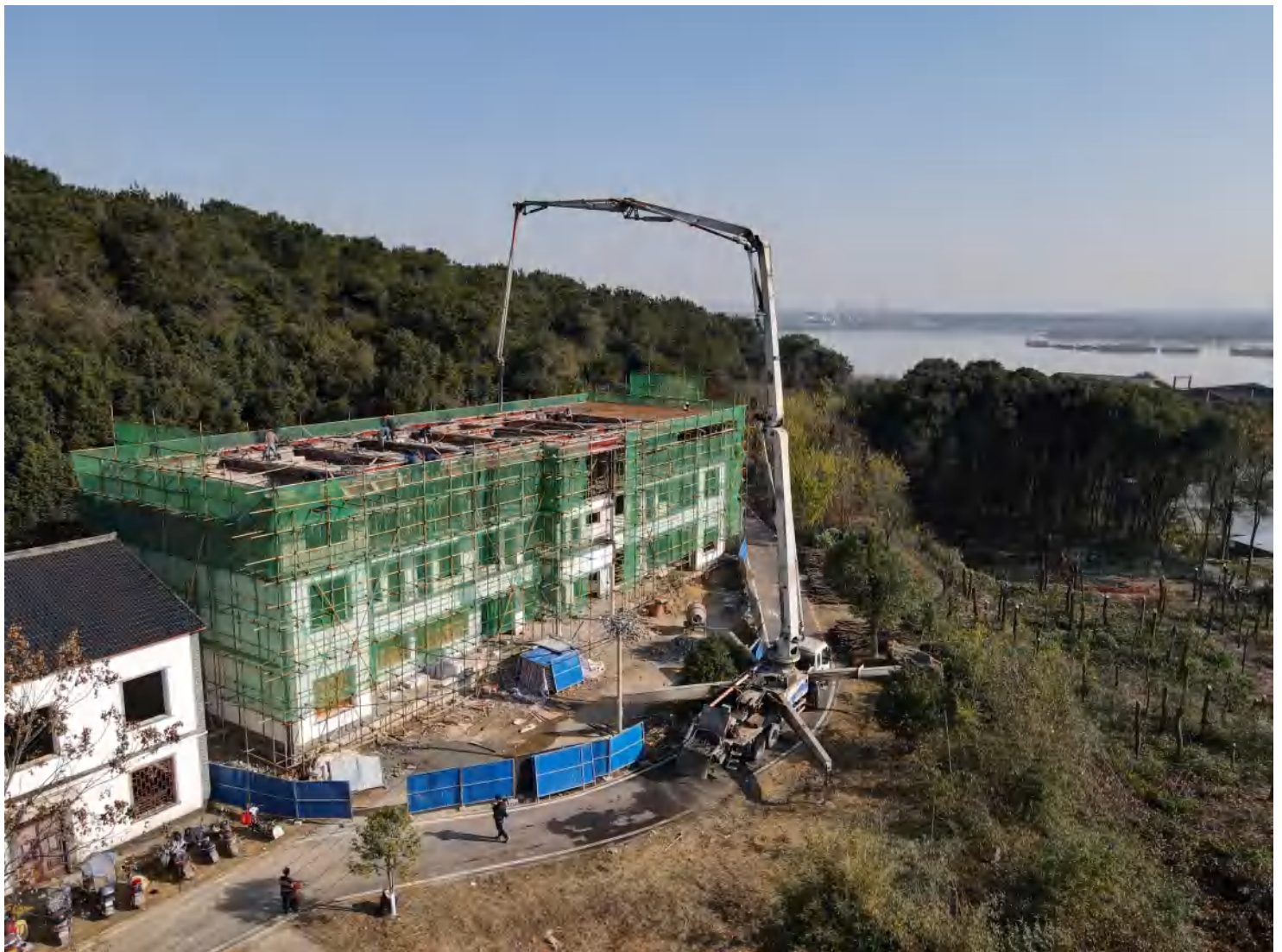
Pouring of Load-Bearing Beams and Columns, December 2021
