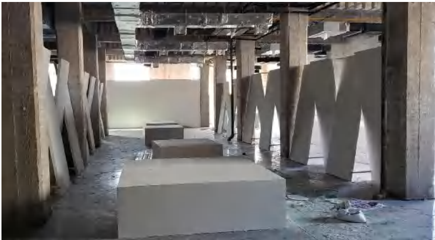
Under Construction, November 2019
