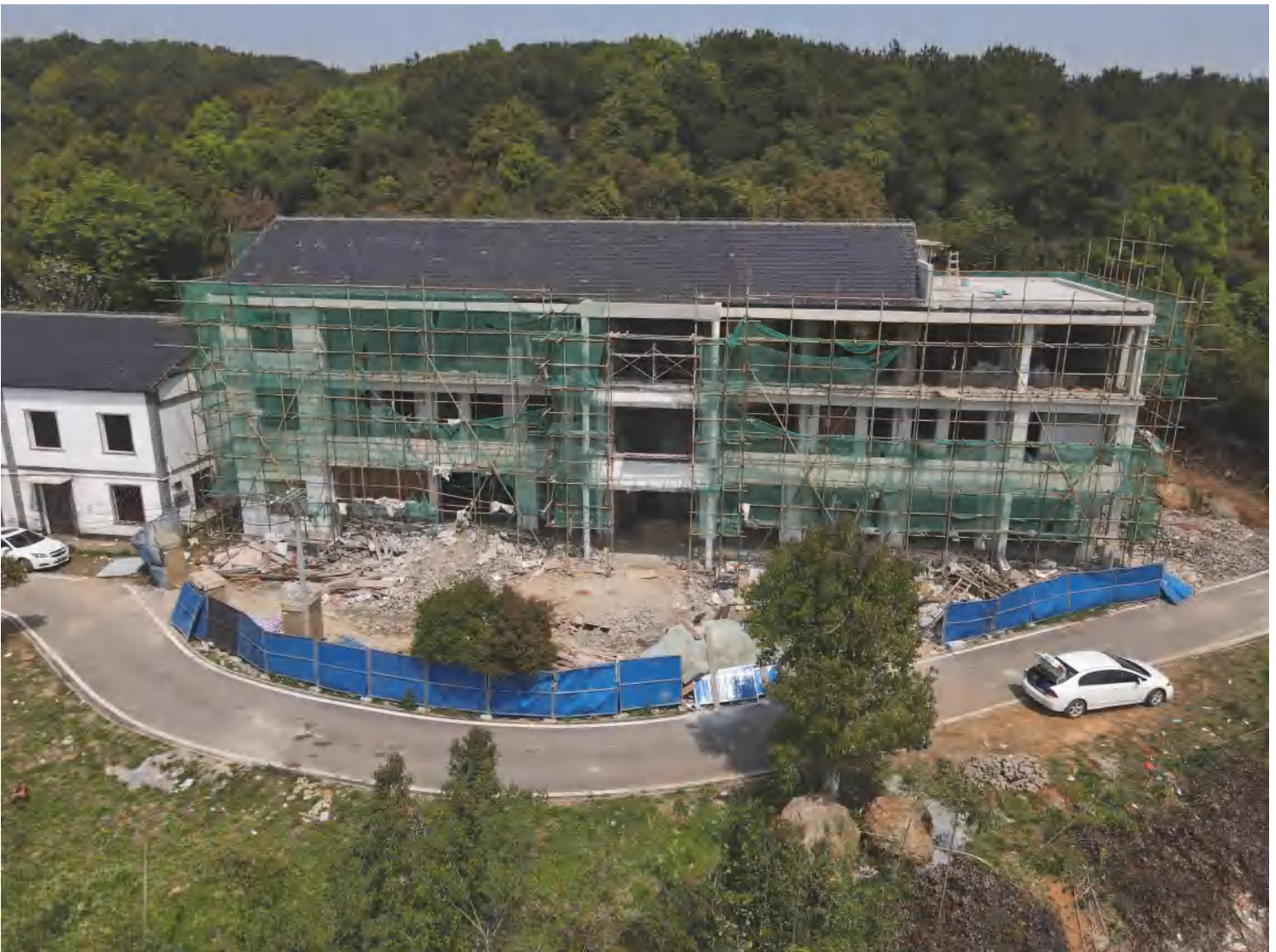
Reinforcement of Building Structure Complete, April 2022
