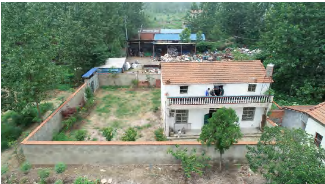
The Original Appearance of the House, June 2020
