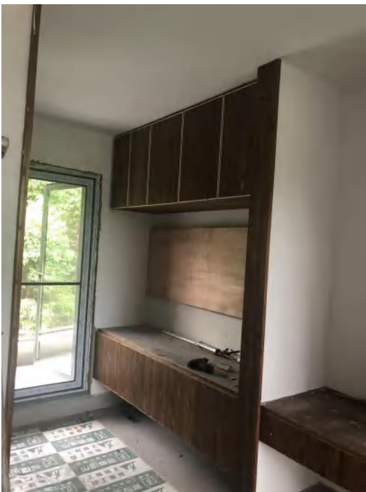
Guest Room is Under Construction, April 2022
