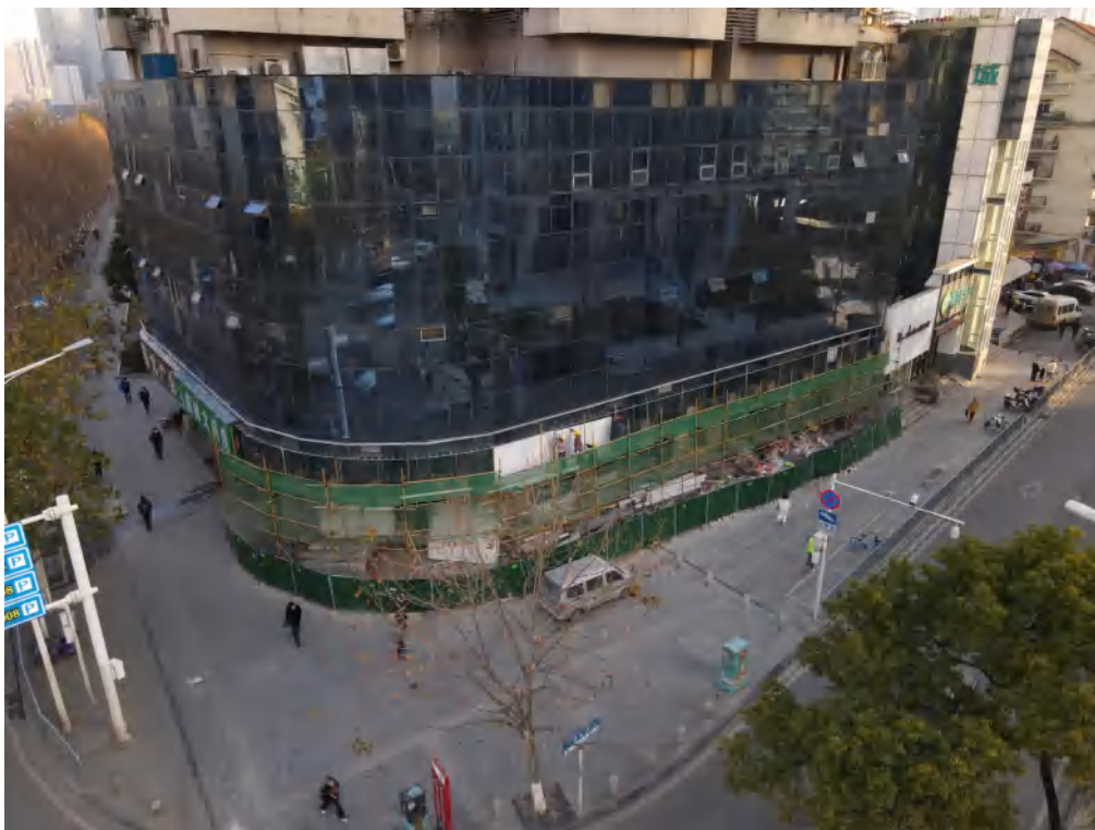
Building Exterior During Construction, February 2022
