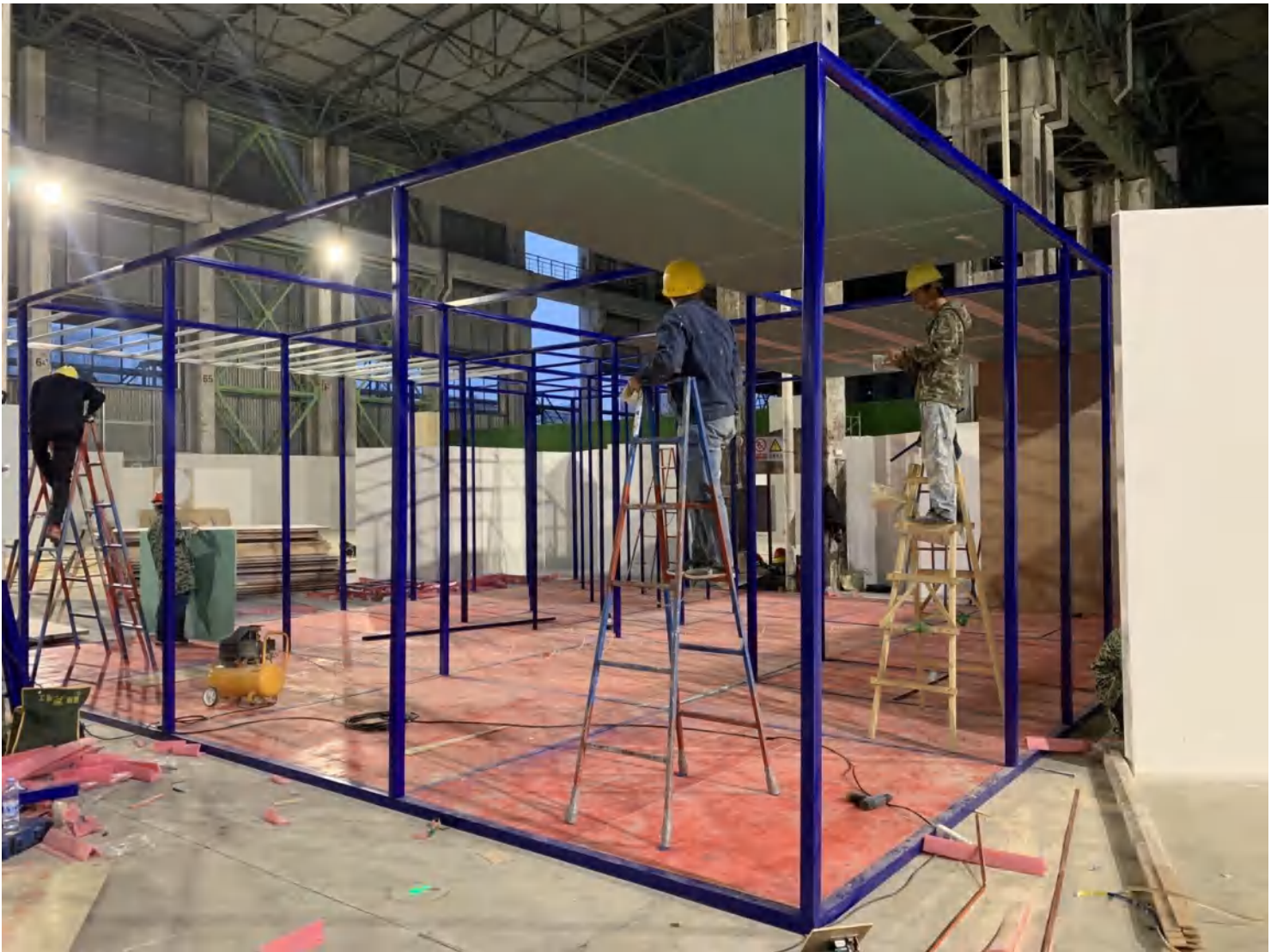
Structural Construction, November 2021
