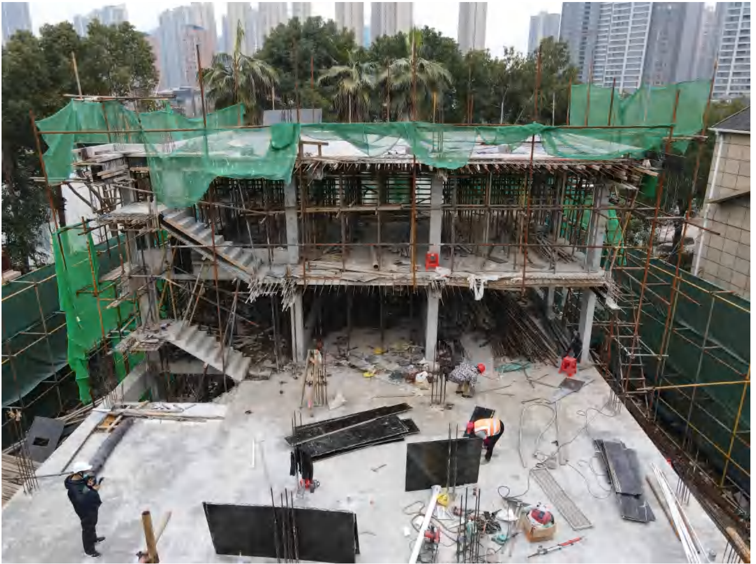
Under Construction, February 2022
