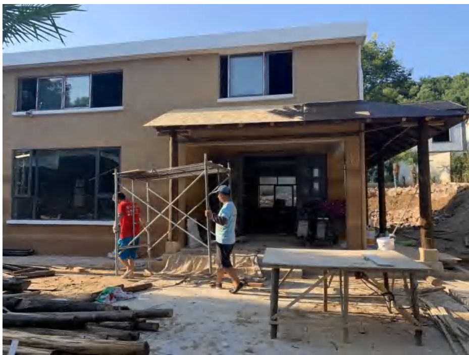
Under Construction, January 2022
