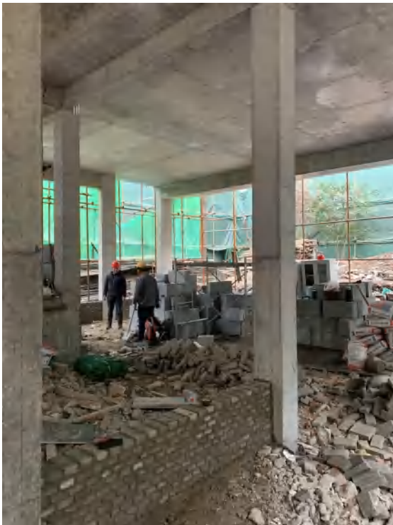
Under Construction, February 2022
