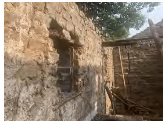
Original Structure of the House October 2021
