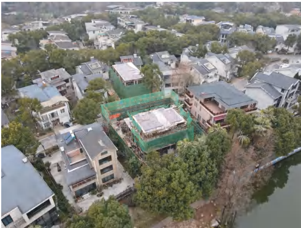
Building Exterior During Construction, February 2022
