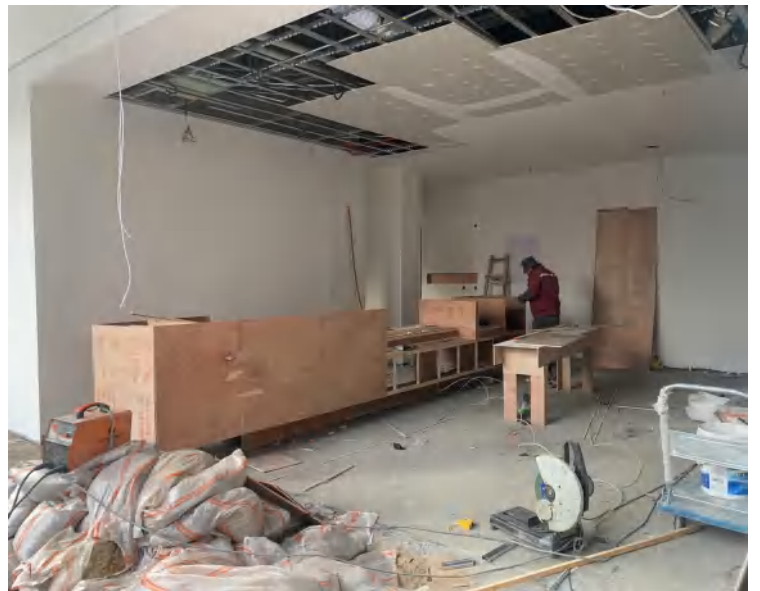
Construction Process, February 2022
