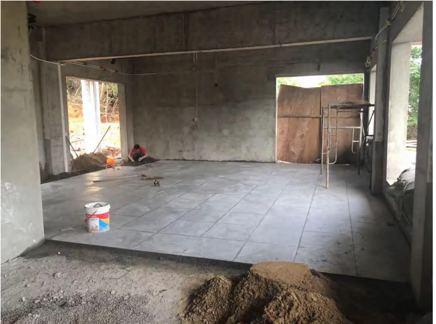
Restaurant is Under Construction, April 2022
