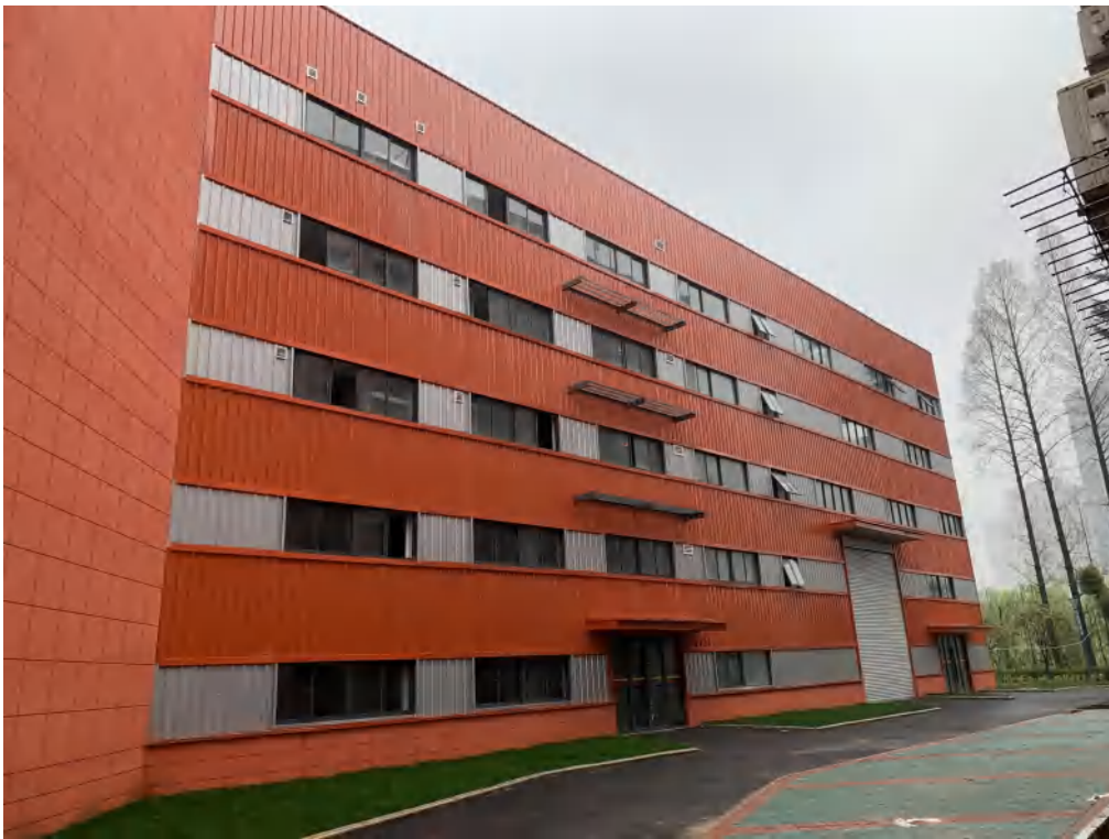
Building Facade, April 2021
