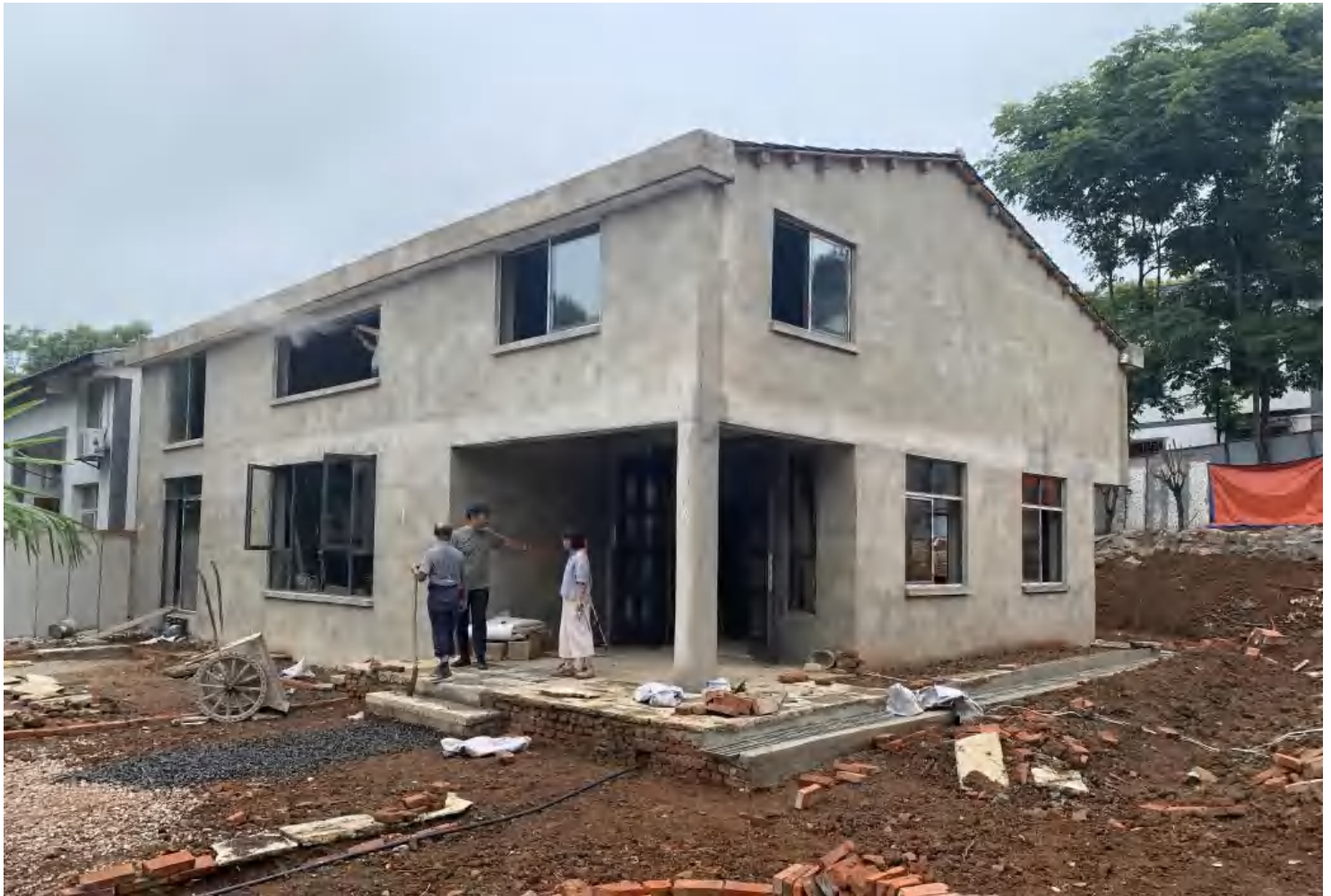
Under Construction, October 2021
