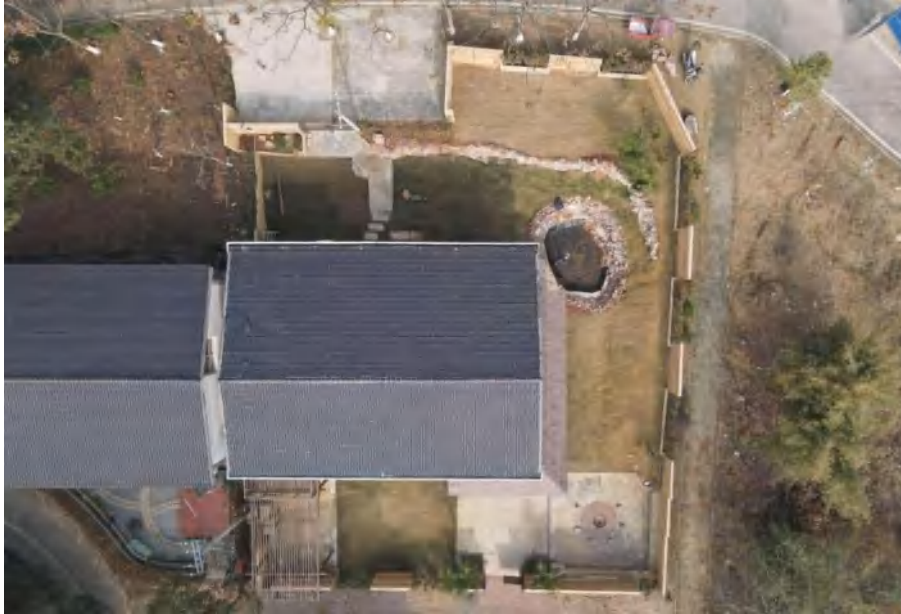
Figure 5-71. Aerial view of Building A(Source: photographed by the author)
