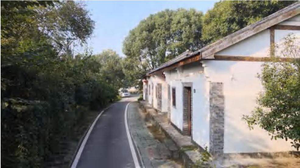
Figure 5-11. Buildings A&B original appearance(Source: photographed by the author)
