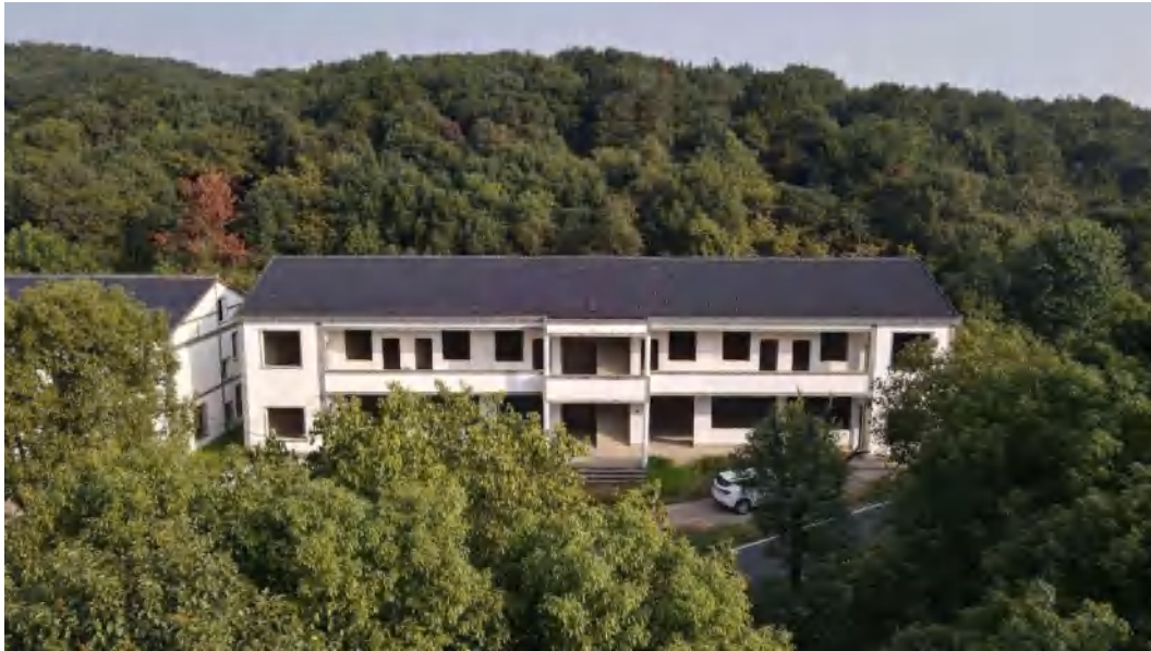
Figure 5-13. Building D original appearance(Source: photographed by the author)
