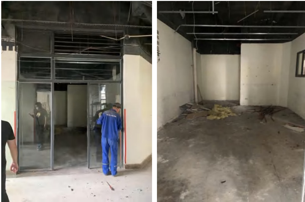
Demolition stage( Source: photographed by the author)
