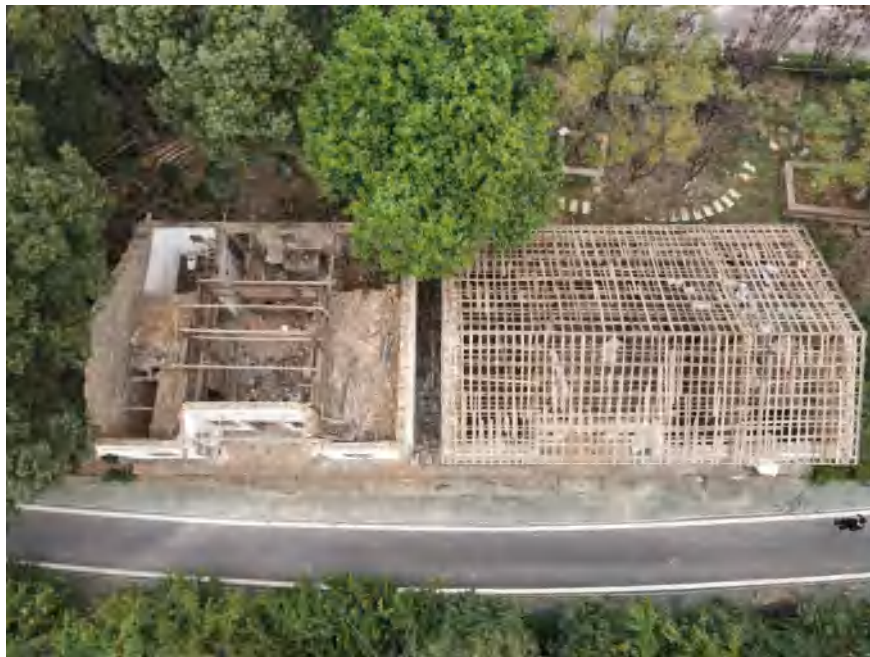
Figure 5-62. Building A&B destruction process(Source: photographed by the author)
