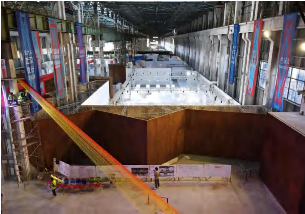
During the construction( Source: photographed by the author)
