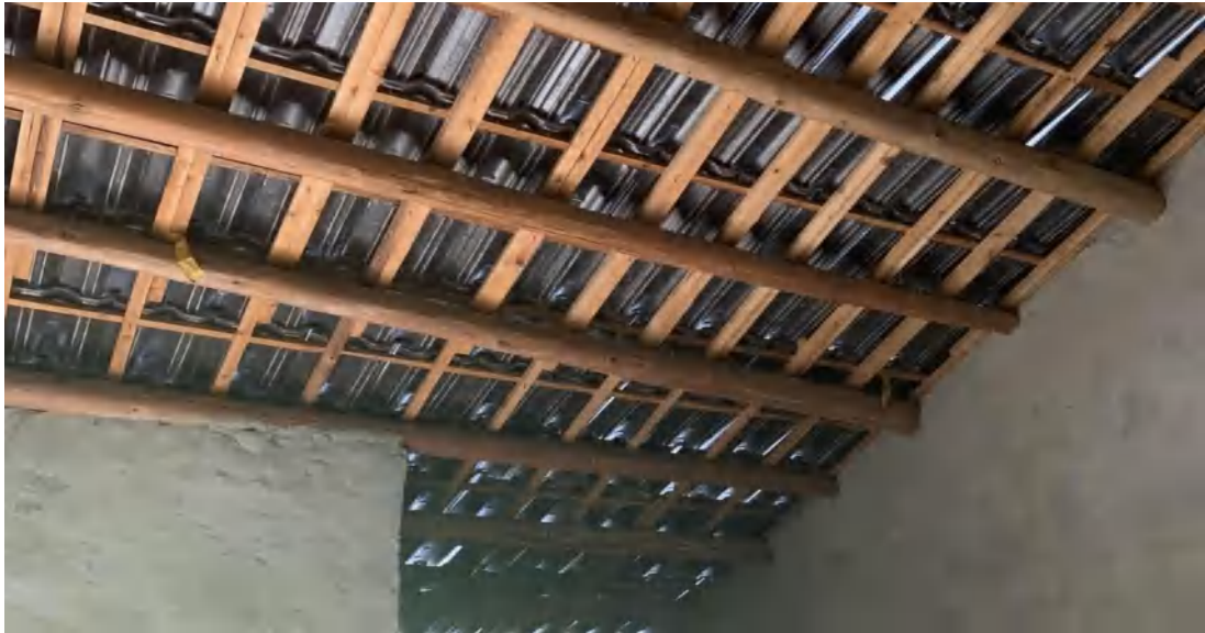
Figure 5-28. Wooden roof of the original building(Source: photographed by the author)
