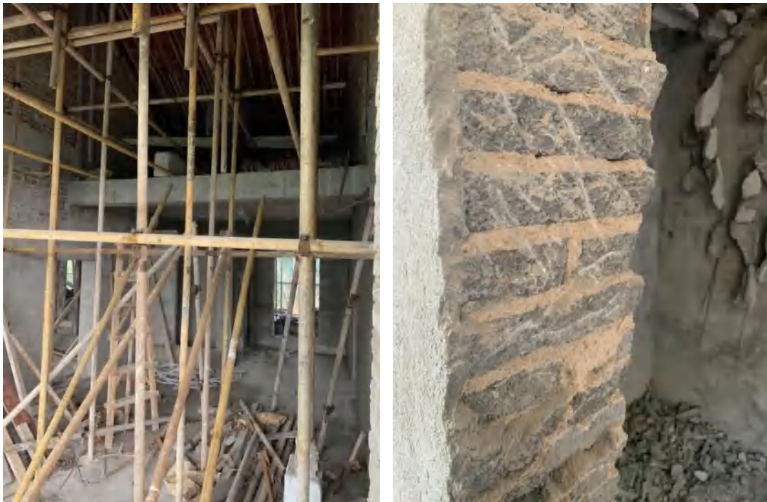
Figure 5-24. Demolition and reinforcement(Source: photographed by the author)
