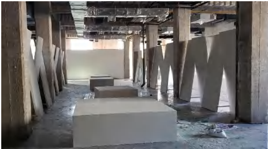
During the construction( Source: photographed by the author)
