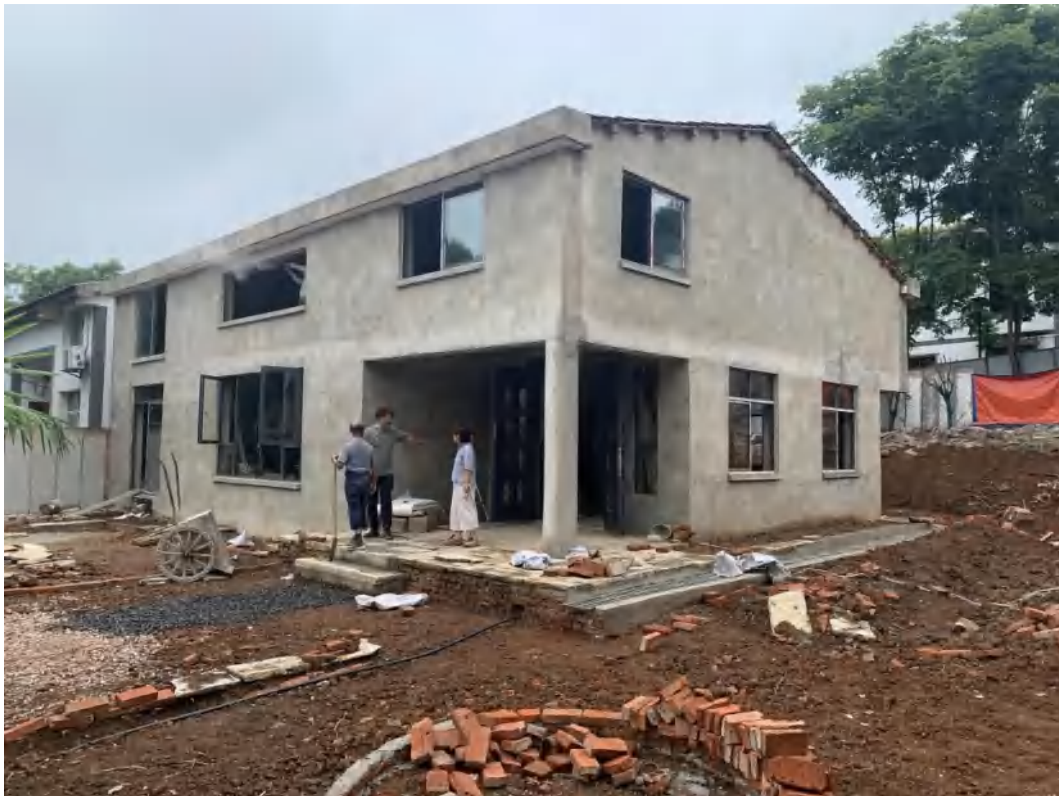
Figure 5-70. Building A early construction(Source: photographed by the author)
