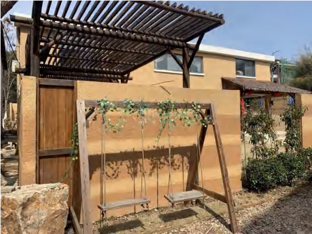
Figure 5-76. Courtyard facade and swing(Source: photographed by the author)
