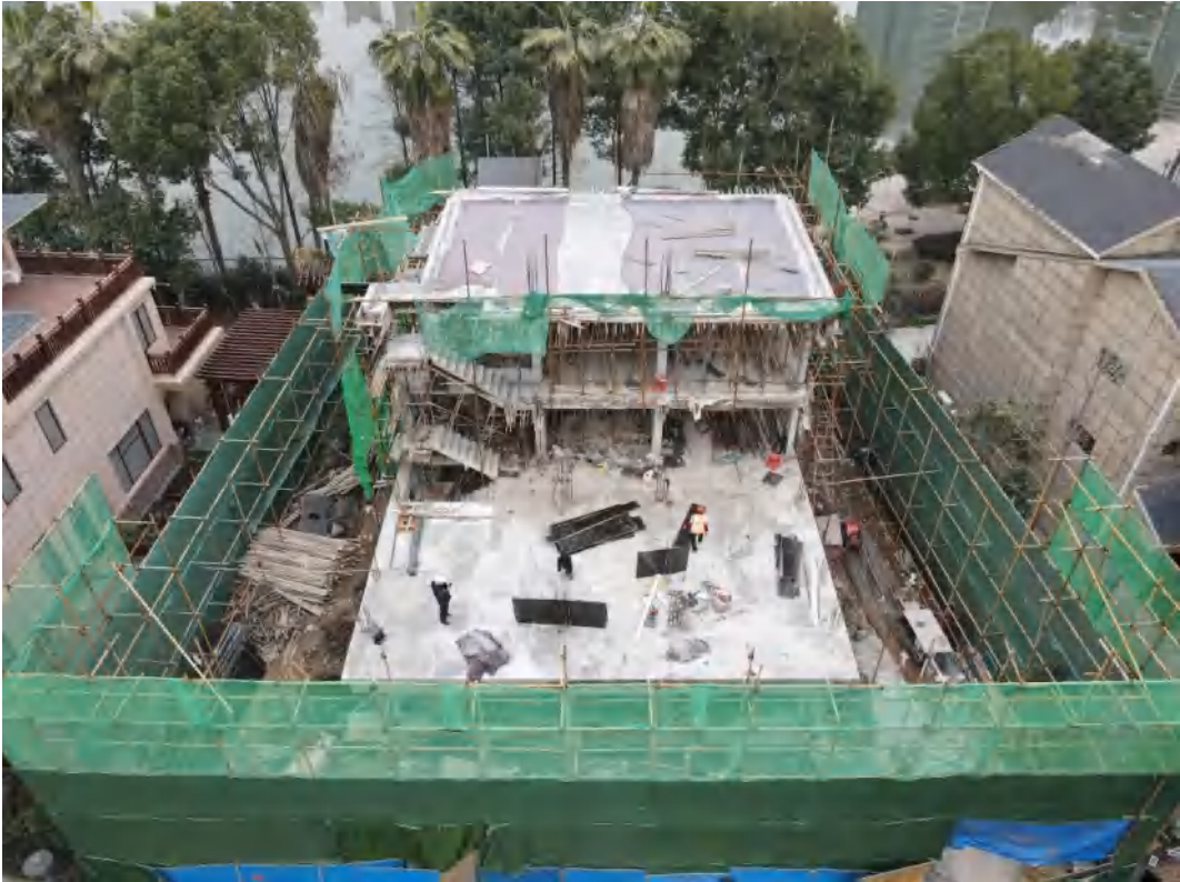
Structural construction( Source: photographed by the author)
