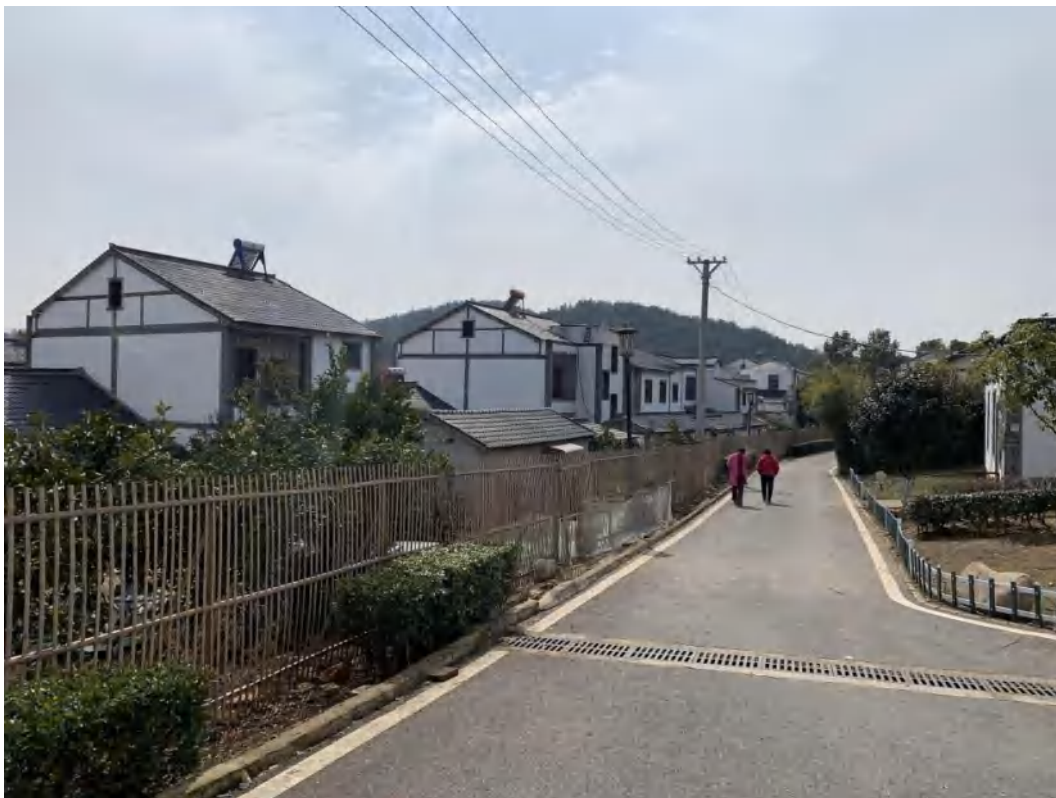
Figure 5-7. Other buildings in Huanghu Village(Source: photographed by the author)
