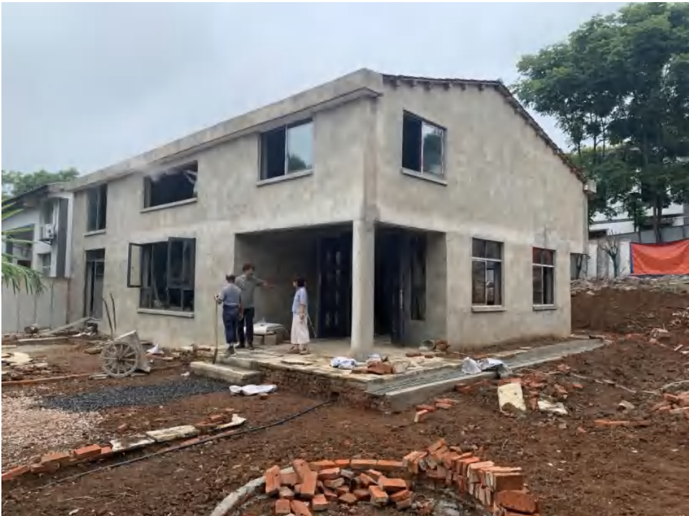
Figure 5-12. Building C is under construction(Source: photographed by the author)
