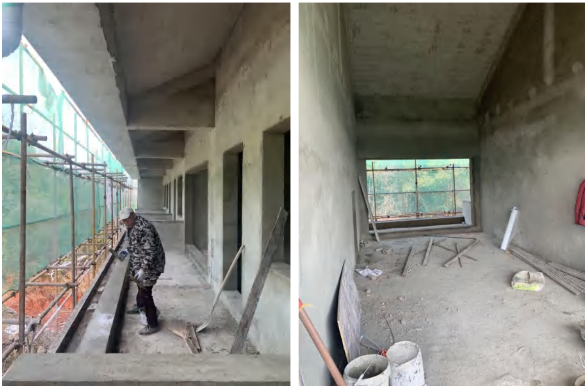
Figure 5-56. Room balcony and window(Source: author's drawing)
