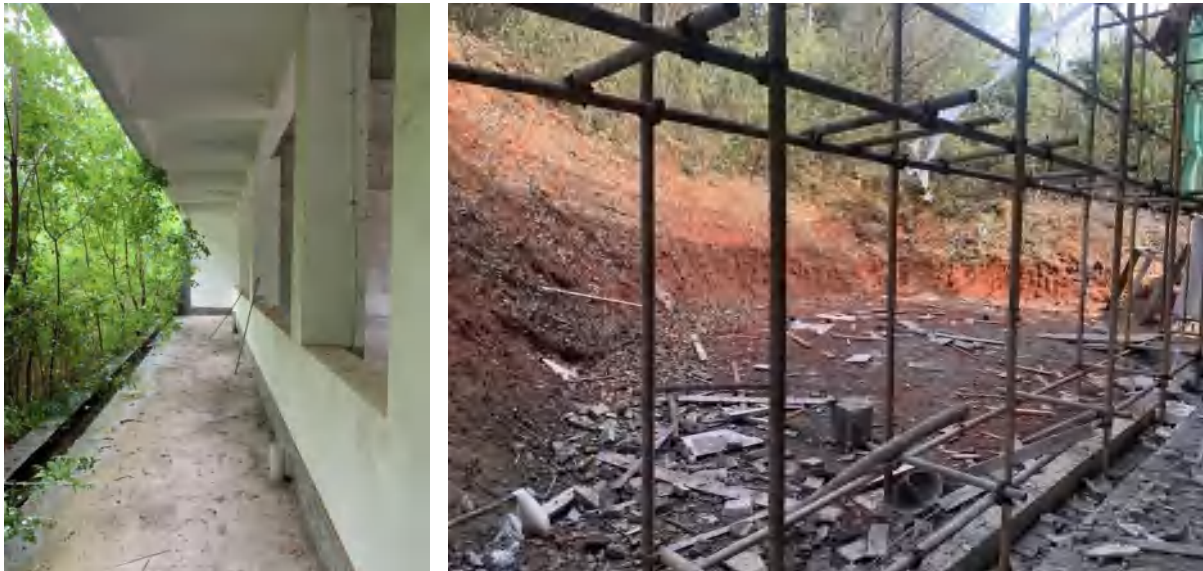
Figure 5-38. Comparison before and after construction(Source: author's drawing)
