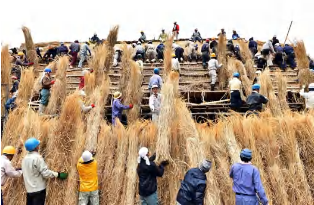
Figure 3-10. Thatched roof(Source: Shirakawa Village Official Website)
