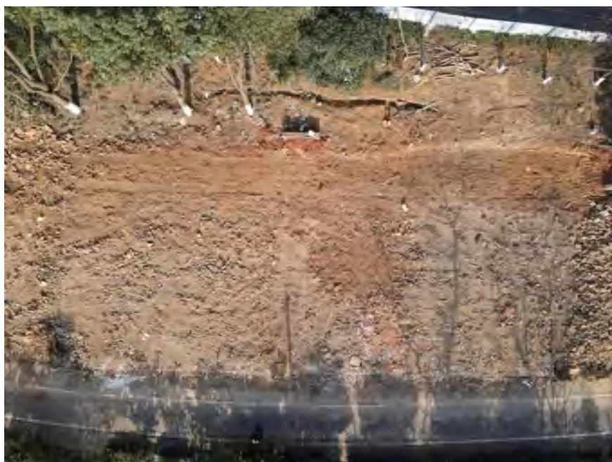
Figure 5-63. Building A&B demolished(Source: photographed by the author)
