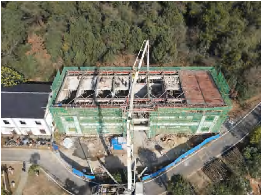
Figure 5-27. Pouring of load-bearing beams and columns(Source: photographed by the author)
