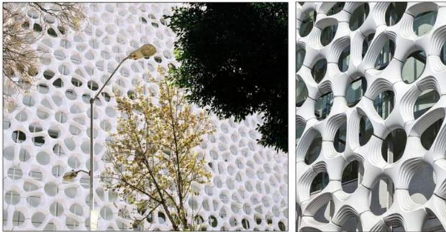
Figure 12. Image The innovative tile material causes a chemical reaction that neutralizes smog. (Image retrieved from http://www.medicaldaily.com/ )
