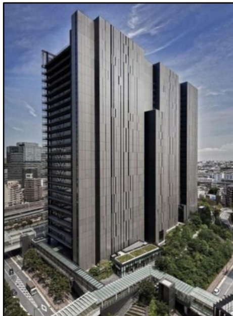
Figure 5. Sony's Osaki Building in Tokyo which is the first building to use the BioSkin exterior system. (Retrieved from: http://www.nikken.co.jp/ )
