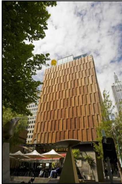
Figure 10. Recycled timber was being used as the building façade of the Council House 2 in Melbourne. (Image retrieved from http://architectuul.com/architecture/ )
