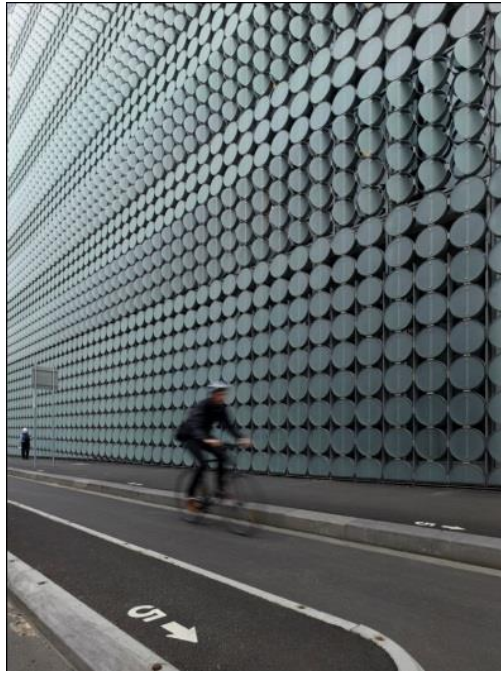
Figure 13. The circular glass panels on RMIT's Design Hub building will soon be replaced with photovoltaic panels that generate solar power. (Image retrieved from: https://architectureau.com/ )
