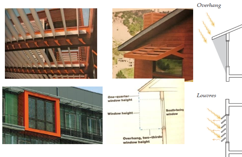
Fig.4.4. Adjustable louvers are used for shading and solar control [15, 23].
