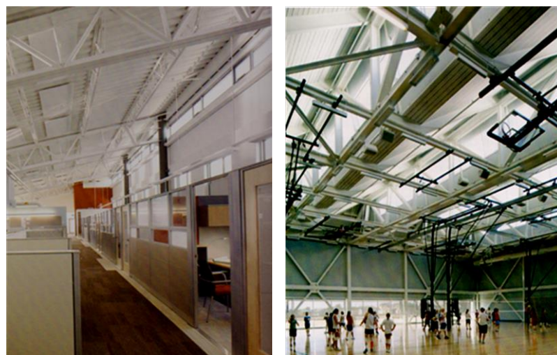
Fig.4.8. Side-lighting in a North Zone (left); Top-lighting in the gymnasium hall (right).
