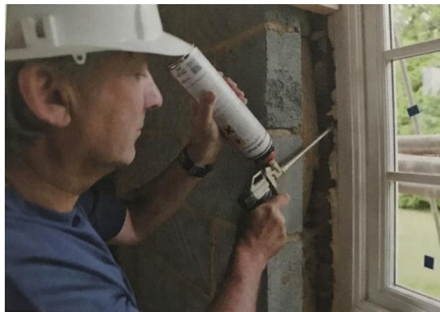
Fig.4.1. Using expansion foam to seal the air gaps [23].
