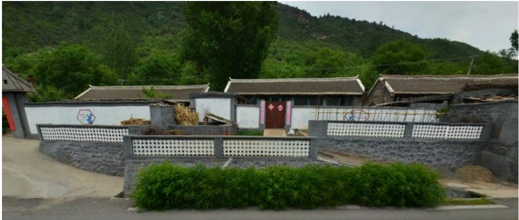
Figure 36. Traditional houses in Beikanzi Village Source: Author
