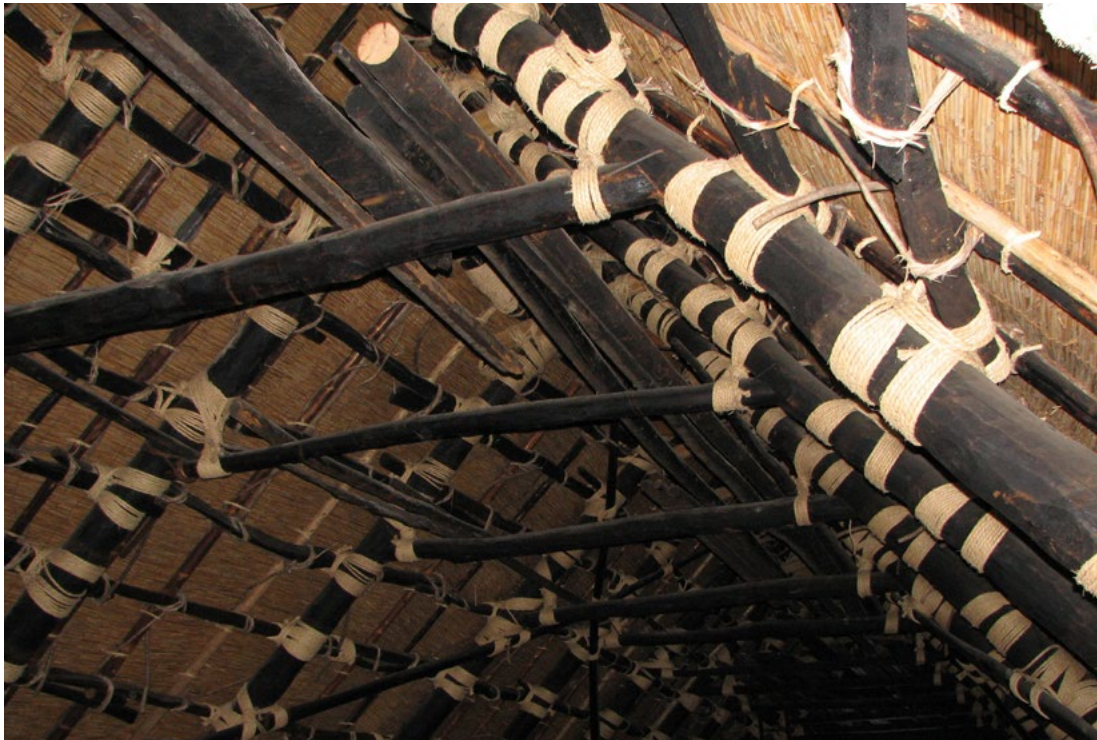
Figure 7. Solid timber roof structures, all tied together by hand with ropes Source: https://upload.wikimedia.org/wikipedia/commons/7/73/Gassho-zukuri_farmhouse-03.jpg
