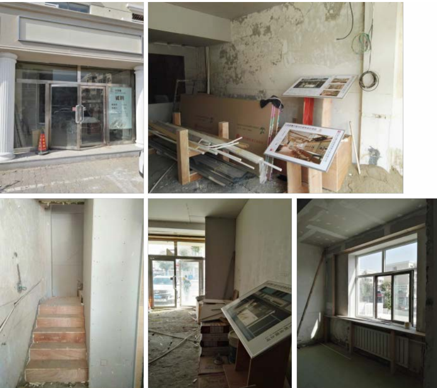
Construction Phase -- this is a reconstruction project
