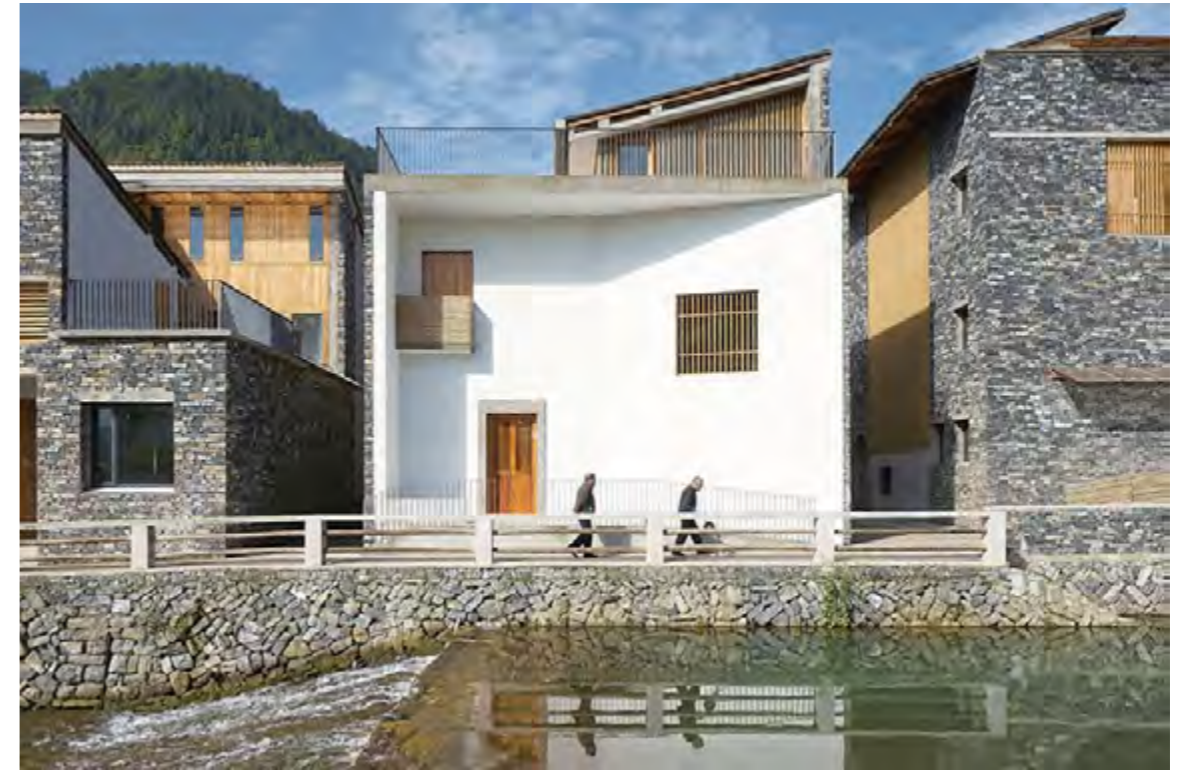
THE RENOVATION PROJECT IN FUYANG
